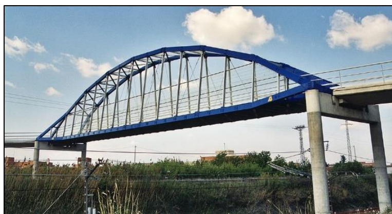
Figure 4: Glass FRP arched pedestrian bridge, 38m x 3m, Lleida, Spain. Railway and vehicle traffic only blocked for three hours during construction [48].
