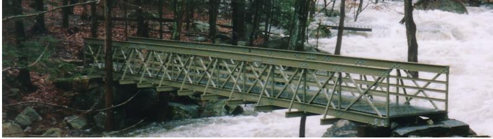
Figure 11: Example of a pedestrian bridge built by Creative Pultrusions. This bridge is in Bear Mountain, New York, and is 62ft x 6ft with a truss design using FRP railings for trusses and FRP decking for the walkway.
