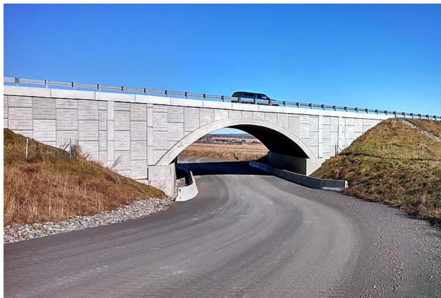
Figure 16: CFFT bridge built by AIT in Augusta, Maine. The bridge uses 22, 15in diameter carbon-fiber tubes to make a span of 54ft, is 55ft wide, and has a rise of 12ft above the concrete abutments to allow enough clearance for traffic once they are placed on the pre-cast concrete foundation.
