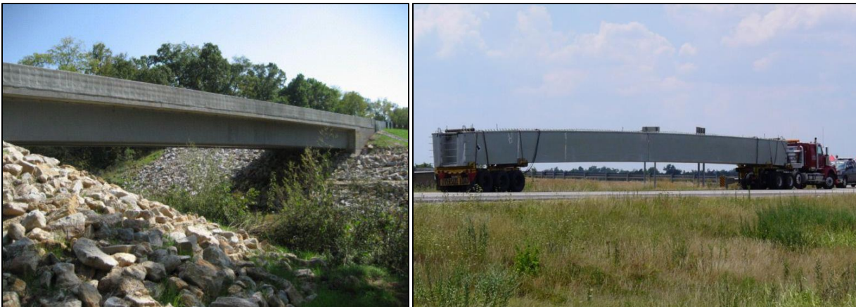
Figure 15: Hillman Composite Beam's HCB bridge near Lockwood, Missouri. The bridge consists of three beams that span 106ft, are 5ft tall, 6ft wide, and support a 30ft 8in wide deck. (Left) Completed bridge. (Right) One of the HCBs being transported on a truck.
