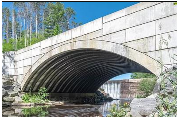
Figure 9: The Perkins Bridge in Belfast, Maine, made with a CFFT and FRP panels. The bridge spans 47ft 7 inches (in), has an 11ft rise, and is 45ft wide. It is made with 16, 15in diameter tubes. Each arch weighed 250 pounds (lbs) before they were filled with concrete [61].
