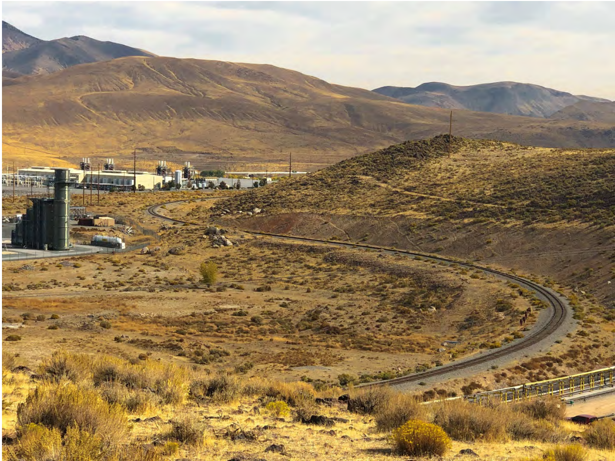
Branch line in the Tahoe-Reno Industrial Center
