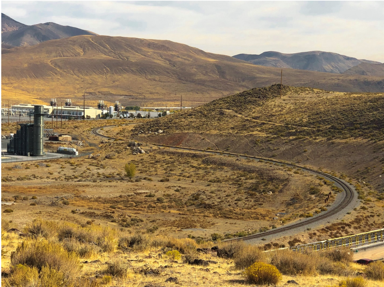
Branch line in the Tahoe-Reno Industrial Center
