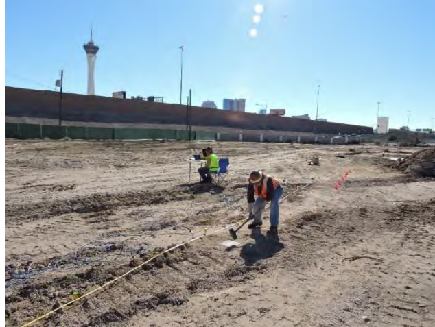
Figure 3.4: Geophysical survey before excavation using MASW method.
