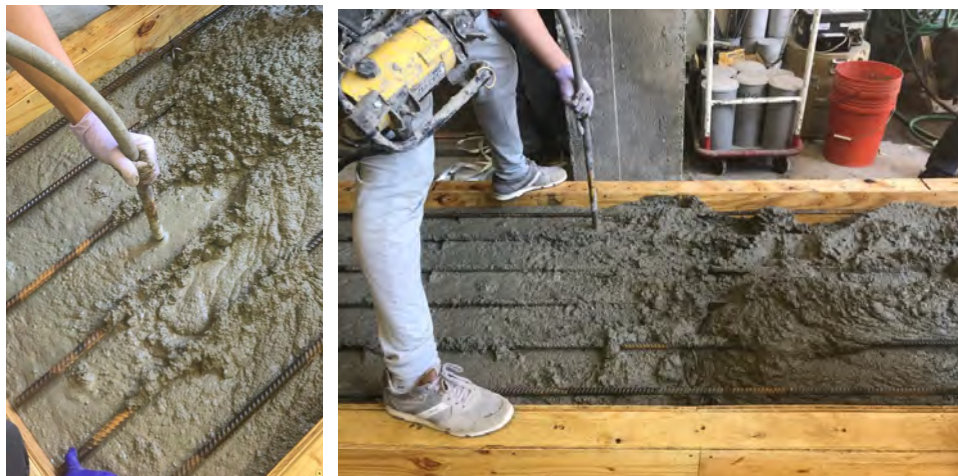
Figure 6.6 Slab concrete before and after vibration
