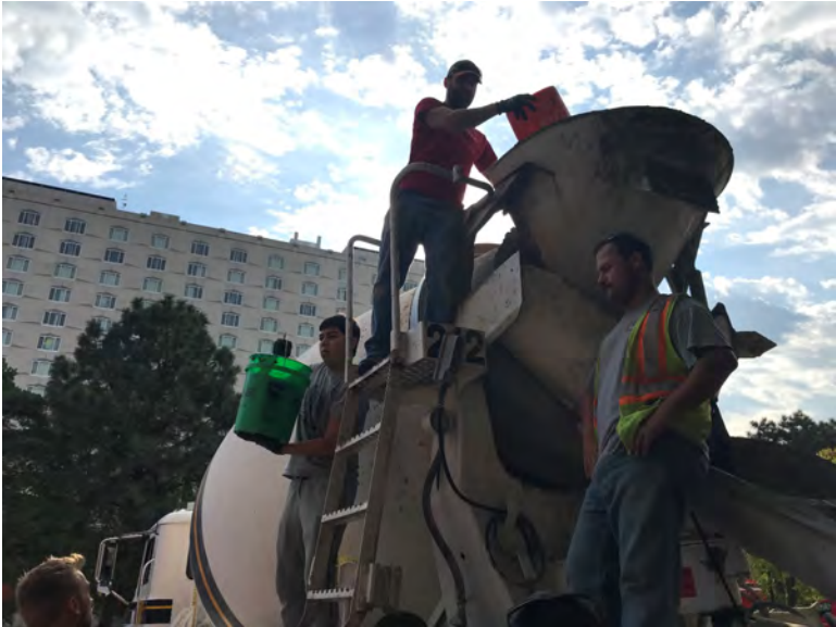
Figure 6.9 Introducing fiber into mixing truck
