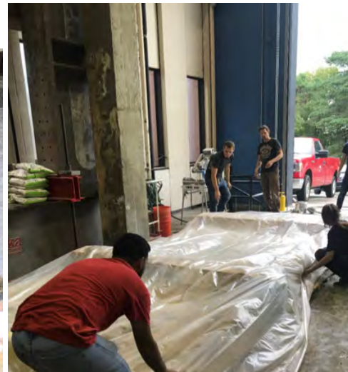
Burlap and plastic wrap for curing
