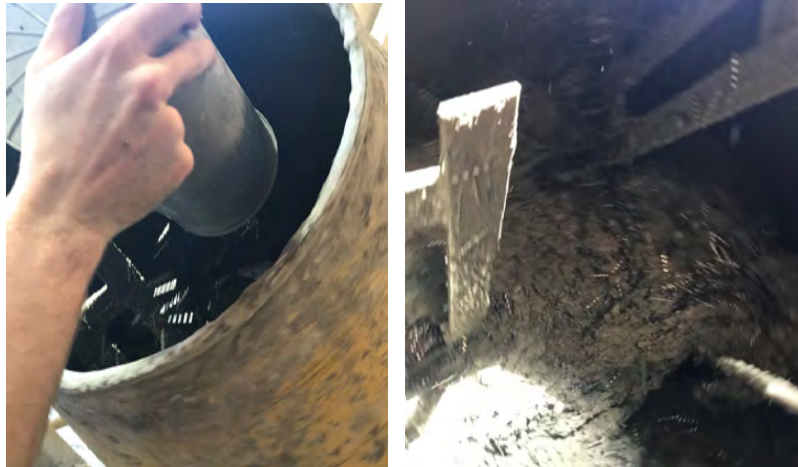
Figure 6.19 Mixing of SHPC for large batch
