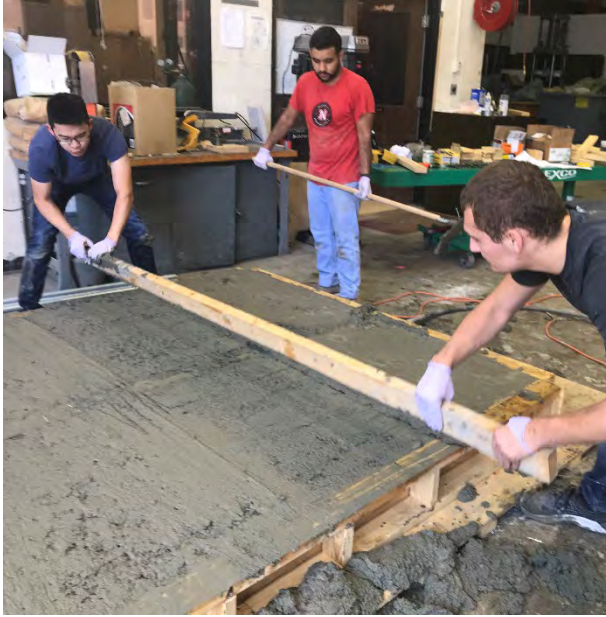
Figure 6.7 Non-FRC slab finishing with screed and bull float
