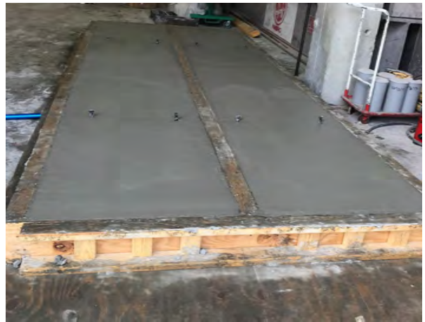
Finished slabs with inserts
