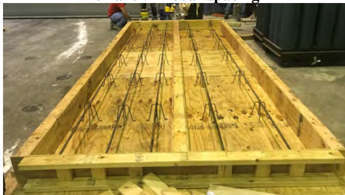
12" and 18" rebar spacing
