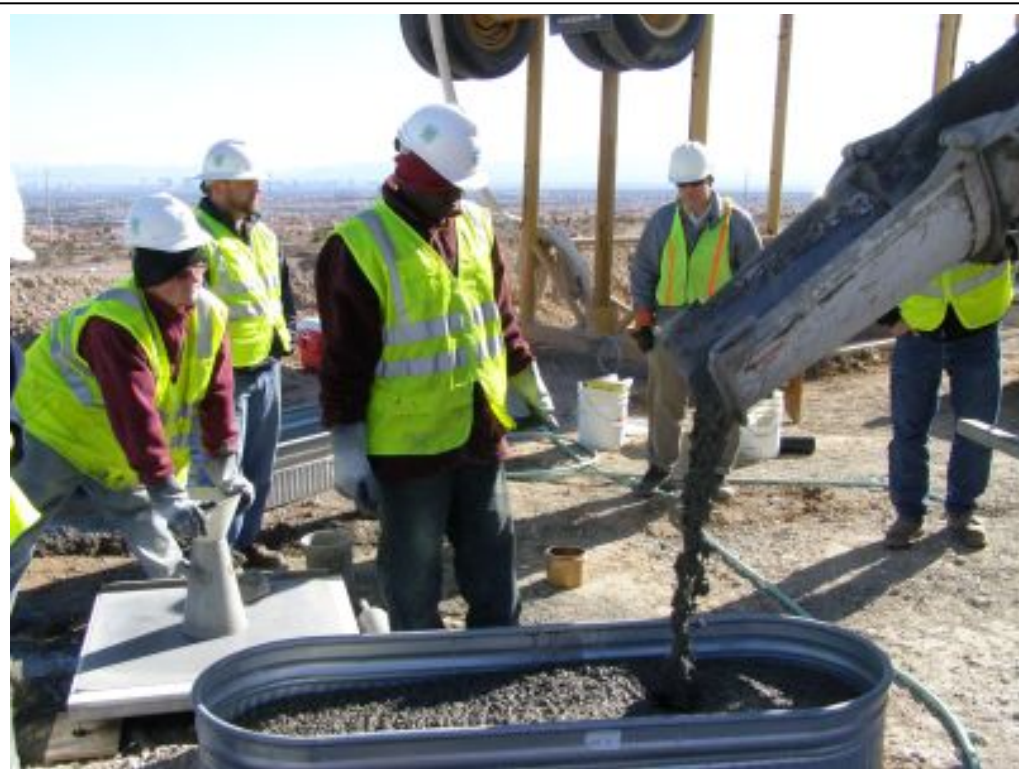
Figure 6.7a: Sample collection of SCC before pumping
