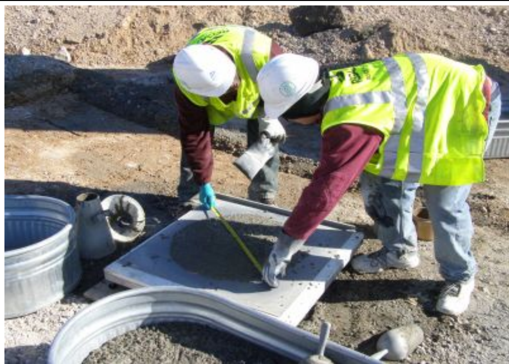
Figure 6.8c: Slump flow test (continued)
