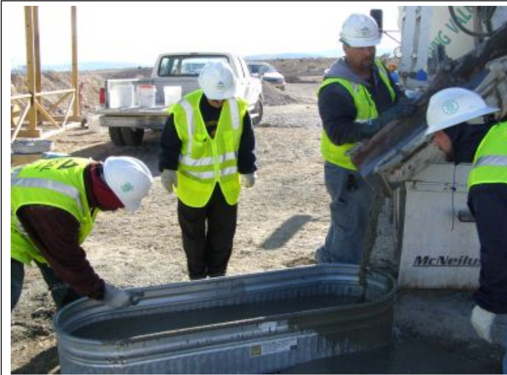
Figure 6.7b: Sample collection of SCC before pumping (continued)
