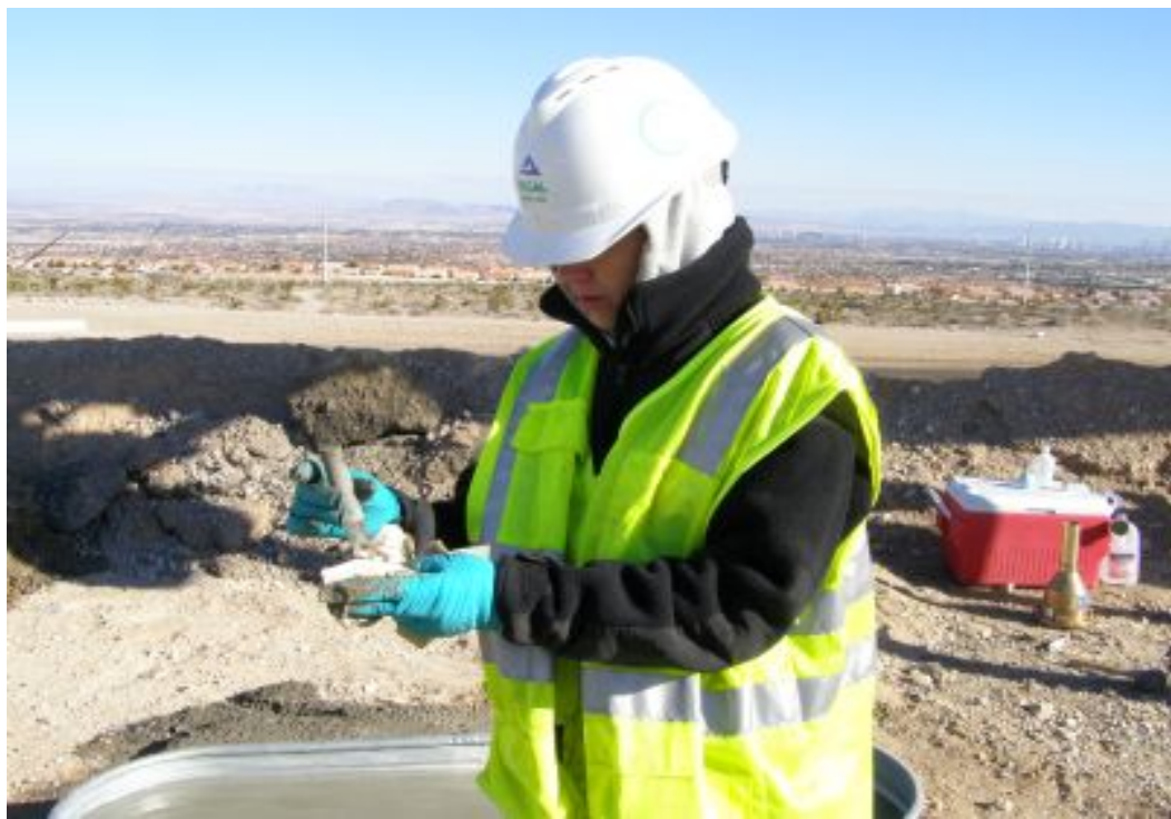
Figure 6.11: Sample collection for air void analysis test
