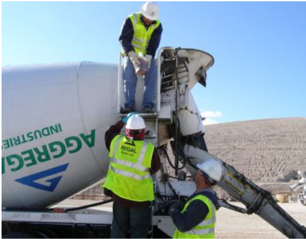
Figure 6.5a: Manual addition of admixture into the fresh concrete
