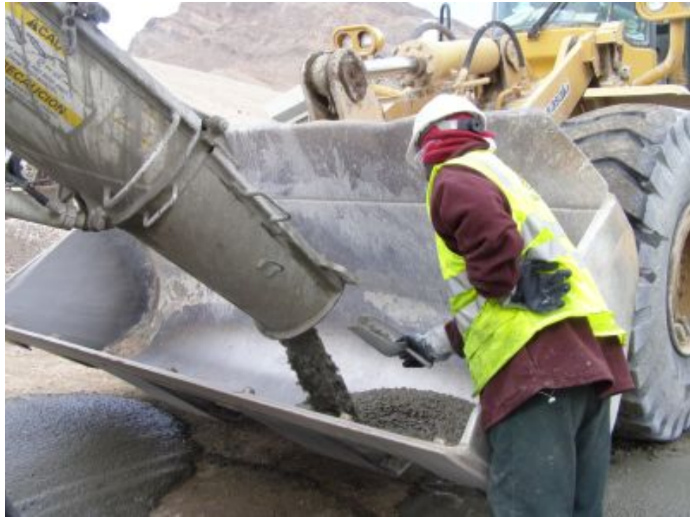
Figure 6.6: Visual inspection of fresh concrete before pumping
