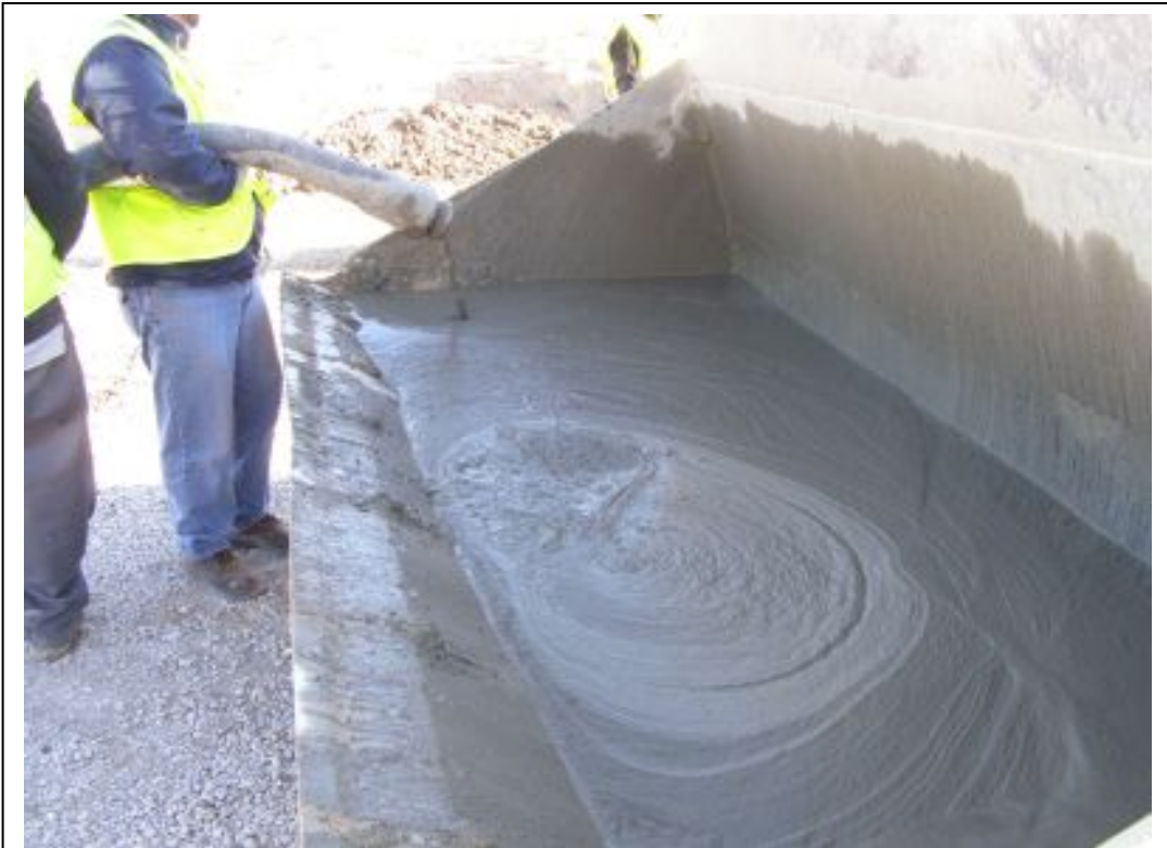
Figure 6.15: Pumping test - lubricating pipes with cement slurry
