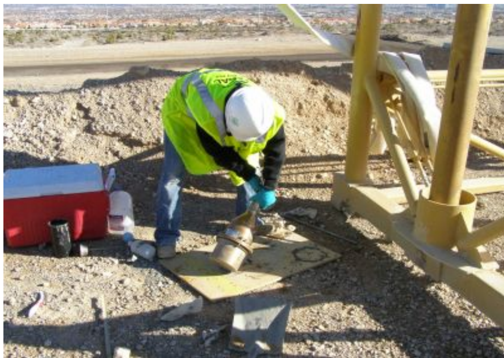
Figure 6.20: Volumetric air content test for post-pumped SCC
