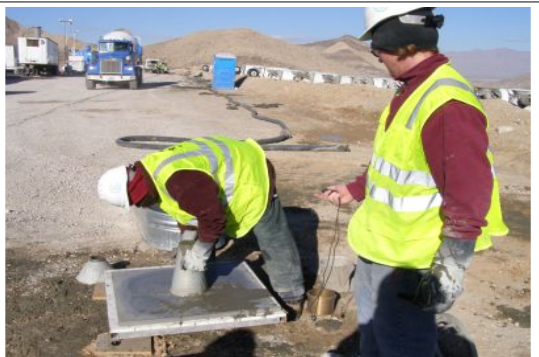
Figure 6.18a: Slump flow and T_{50} tests for post-pumped SCC
