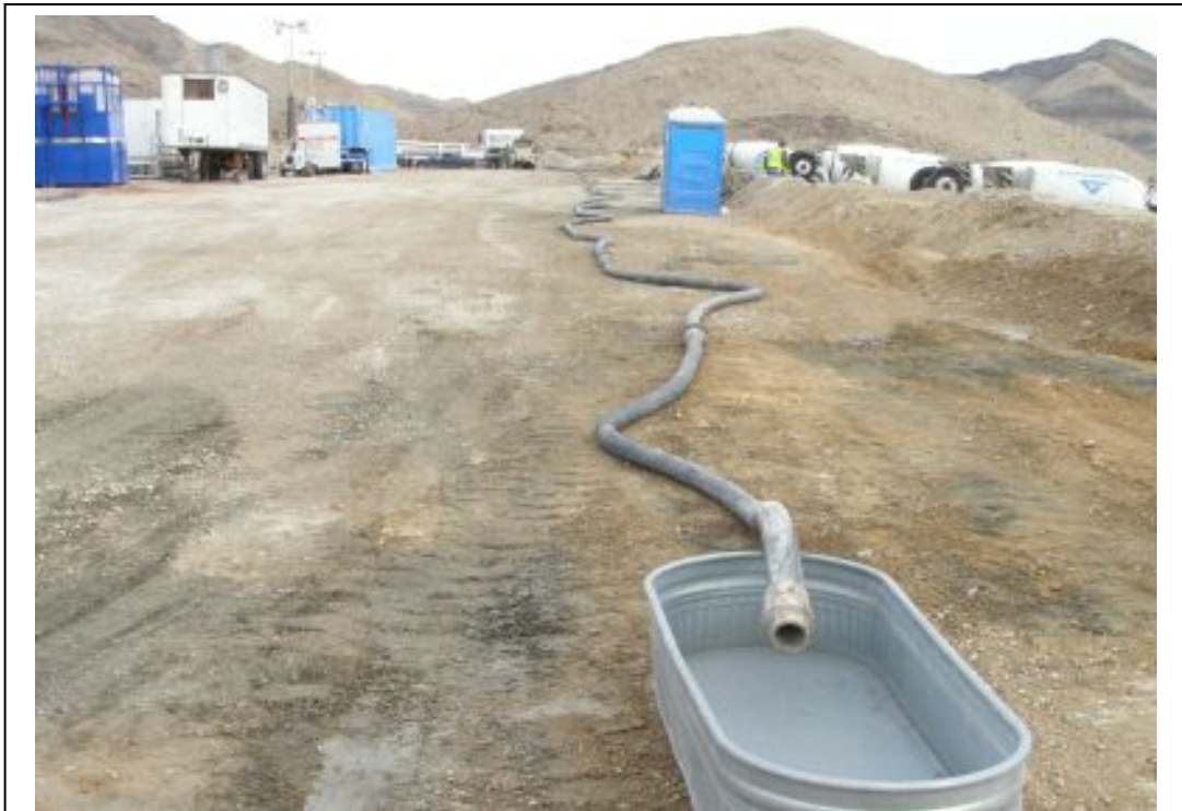
Figure 6.14: Pumping test - set up of pipeline
