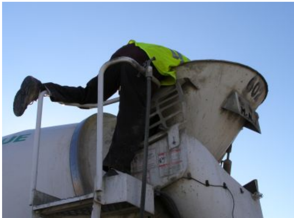
Figure 6.5b: Manual addition of admixture into the fresh concrete (continued)
