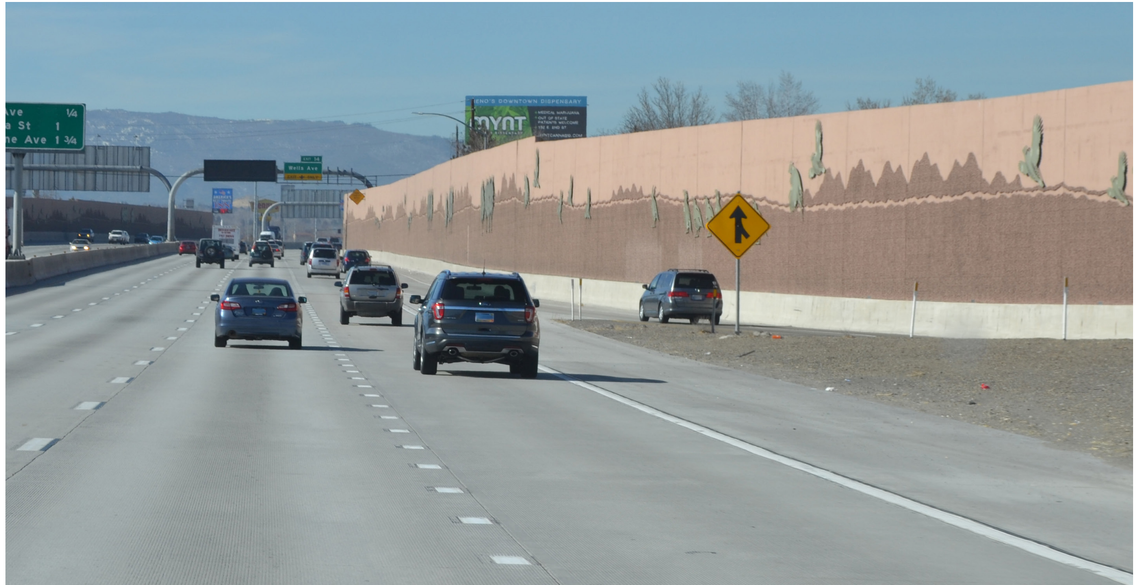
Existing traffic noise barriers at the I-80/Wells Avenue interchange
