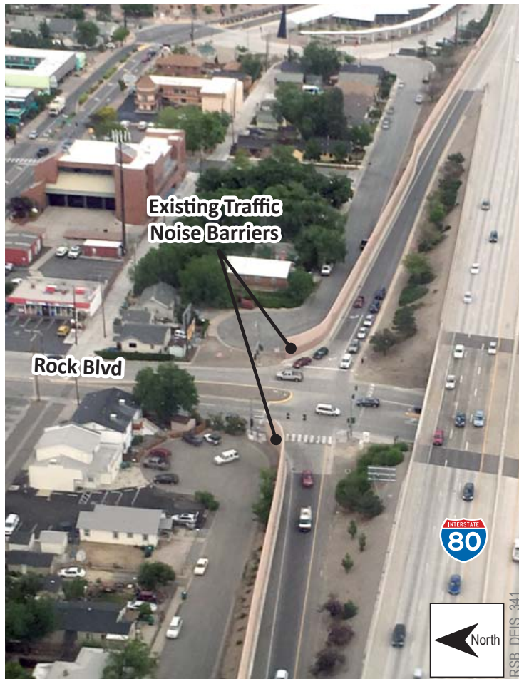
Existing traffic noise barriers at the I-80/Rock Boulevard interchange
