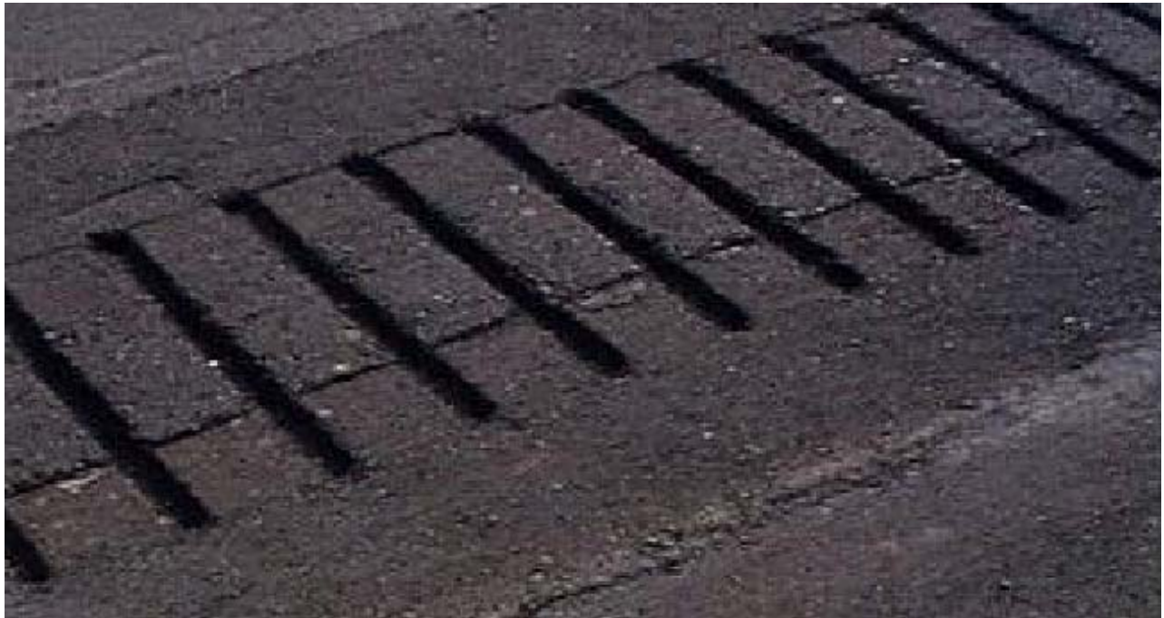
Figure 2: Rolled Rumble Strips
