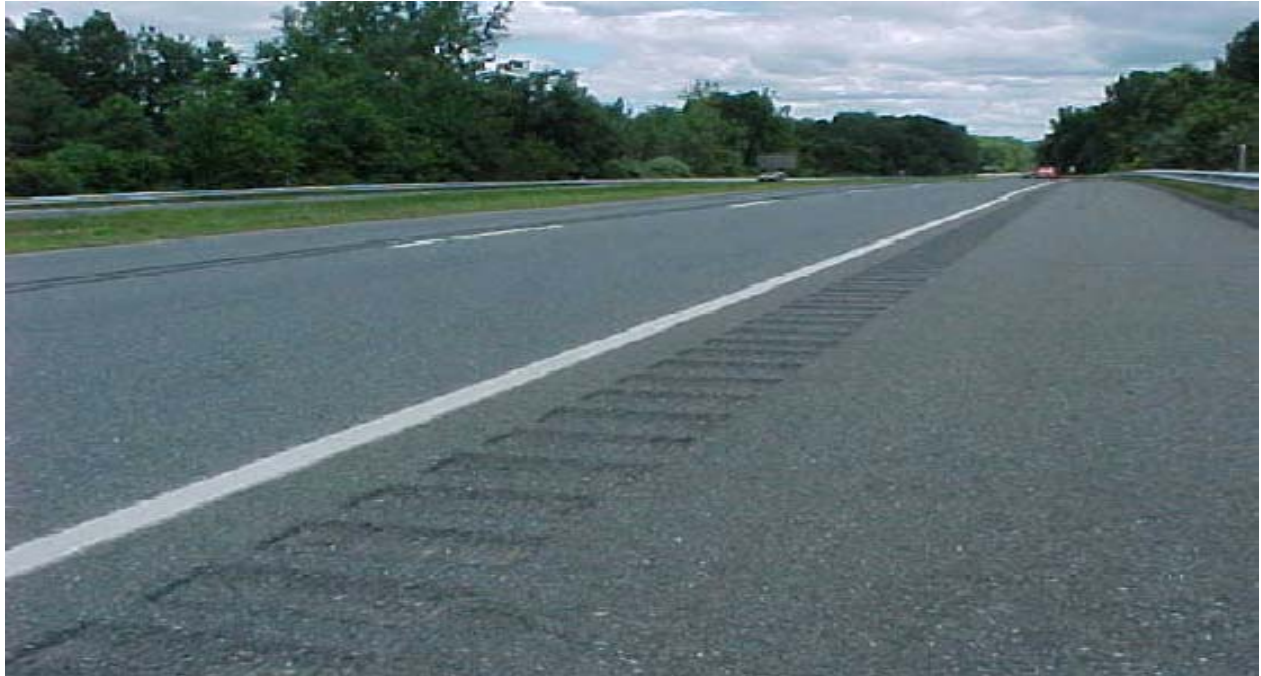
Figure 1: Milled Rumble Strips (Source: http://people.umass.edu/vetri/ThesisProposal.pdf ; Accessed November 2004)
