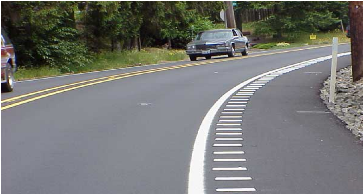
Figure 3: Raised Rumble Strips
