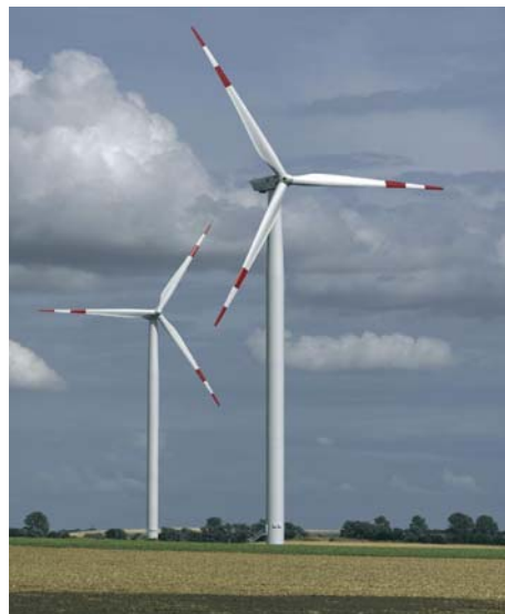
Fig 2.5 Image of a large GE wind turbines with 2 MW output power [10]
