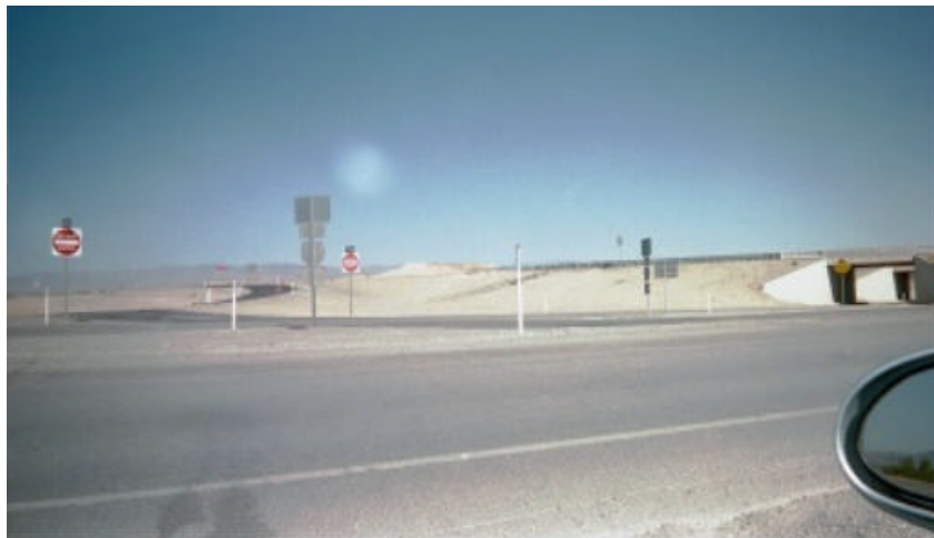
Example #3. Interchange of off Interstate 15 to the Valley of Fire, east of Las Vegas
