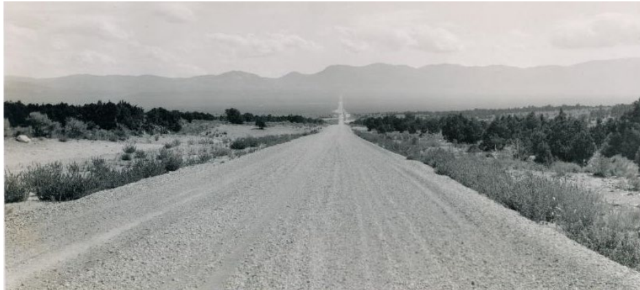
Figure 14. c.1927 photo of the Victory Highway west of Moor, Nevada, showing gravel roadbed. 107
