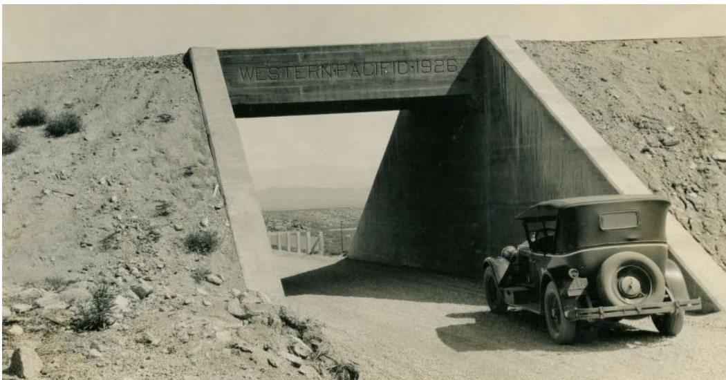
Figure 26. c.1927 image of the railroad underpass at Silver Zone Summit on the Victory Highway. 155
