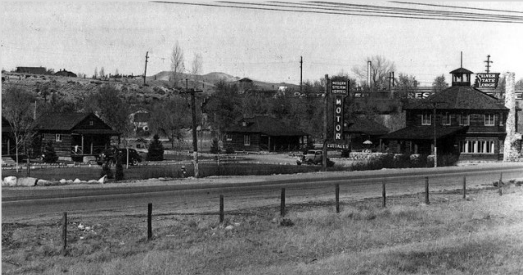
Figure 28. The 1931 Silver State Lodge (nonextant), on a portion of the route cosigned as the Victory Highway and Lincoln Highways, catered to divorce-seekers. 168
