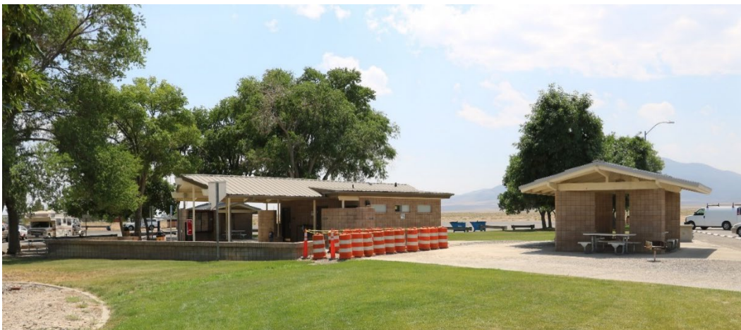
Figure 34. Image of c.1960 rest stop at Valmy, with restrooms at left of image and picnic shelter at right.
