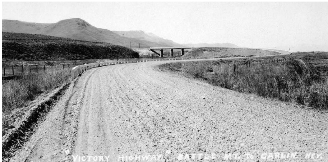
Figure 17. Grade-separation structure on the Victory Highway between Carlin and Battle Mountain, c. 1927. 118
