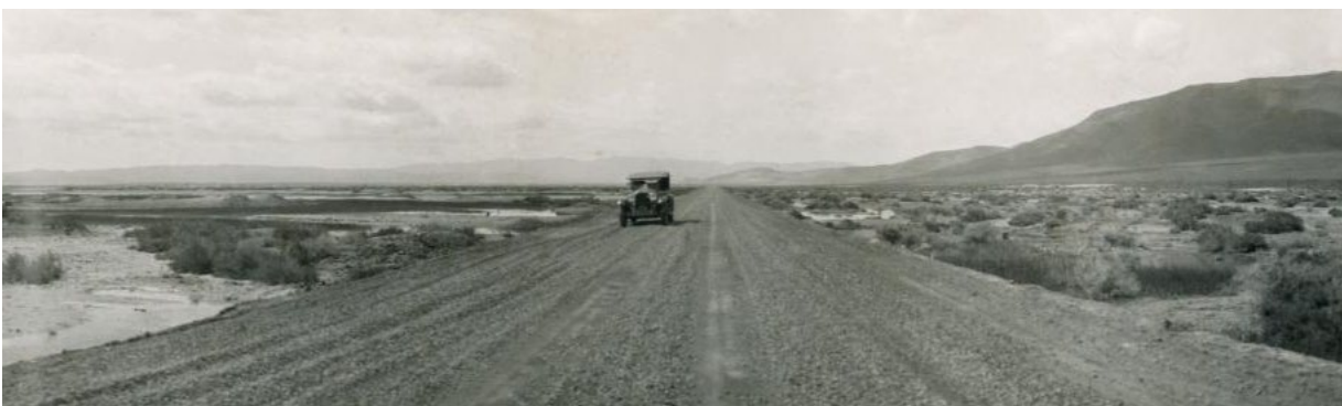
Figure 22. The Victory Highway approximately 3.1 miles west of Wadsworth, c.1927.
