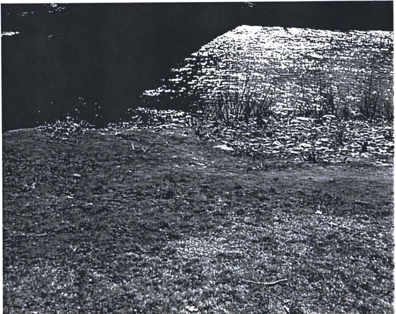
Keystone Bridge – NW Corner (looking south)
