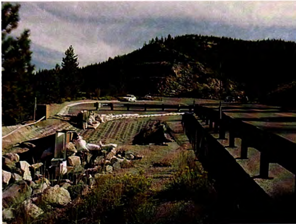
Figure 6.1. NDOT 3, U.S. Highway 50 sediment basin.
