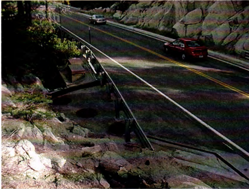
Figure 4.2. Triple-barrel sediment trap at Secret Harbor Creek.
