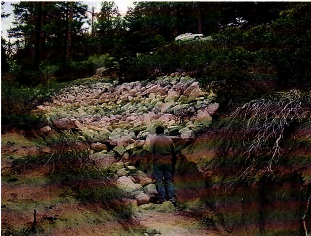
Figure 9.1. Riprap channel terminus on steep hillside below SR 28.
