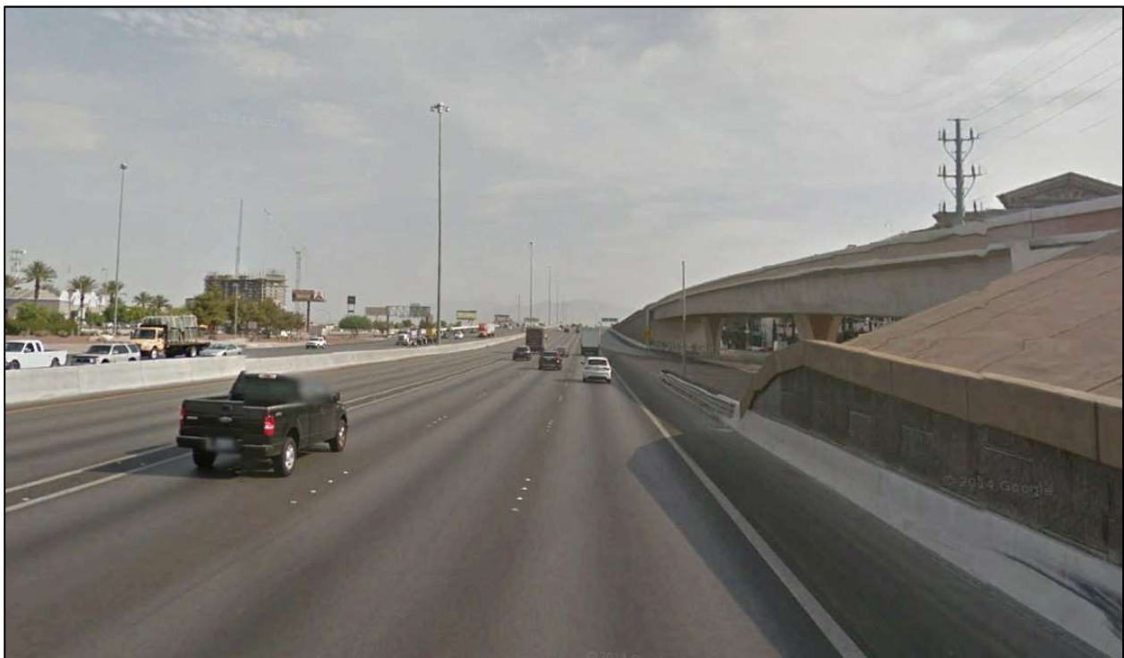
0’ to 2’ inside and outside shoulders with six 11’ lanes (2-11’ HOV and 4-11’ GP lanes)
