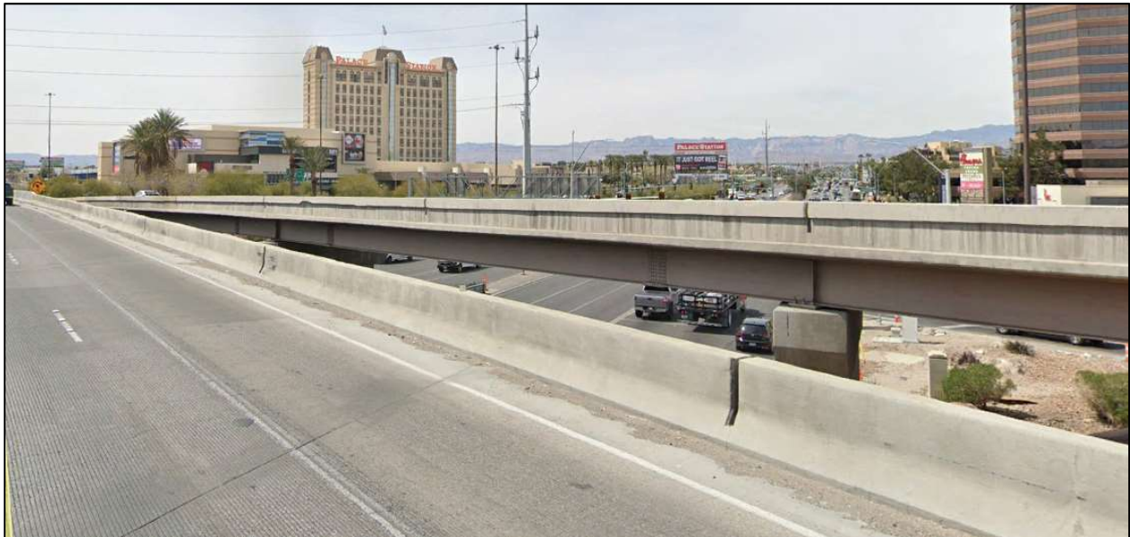
Not enough bridge width for six 11' lanes (2-11' HOV and 4-11' GP lanes)
