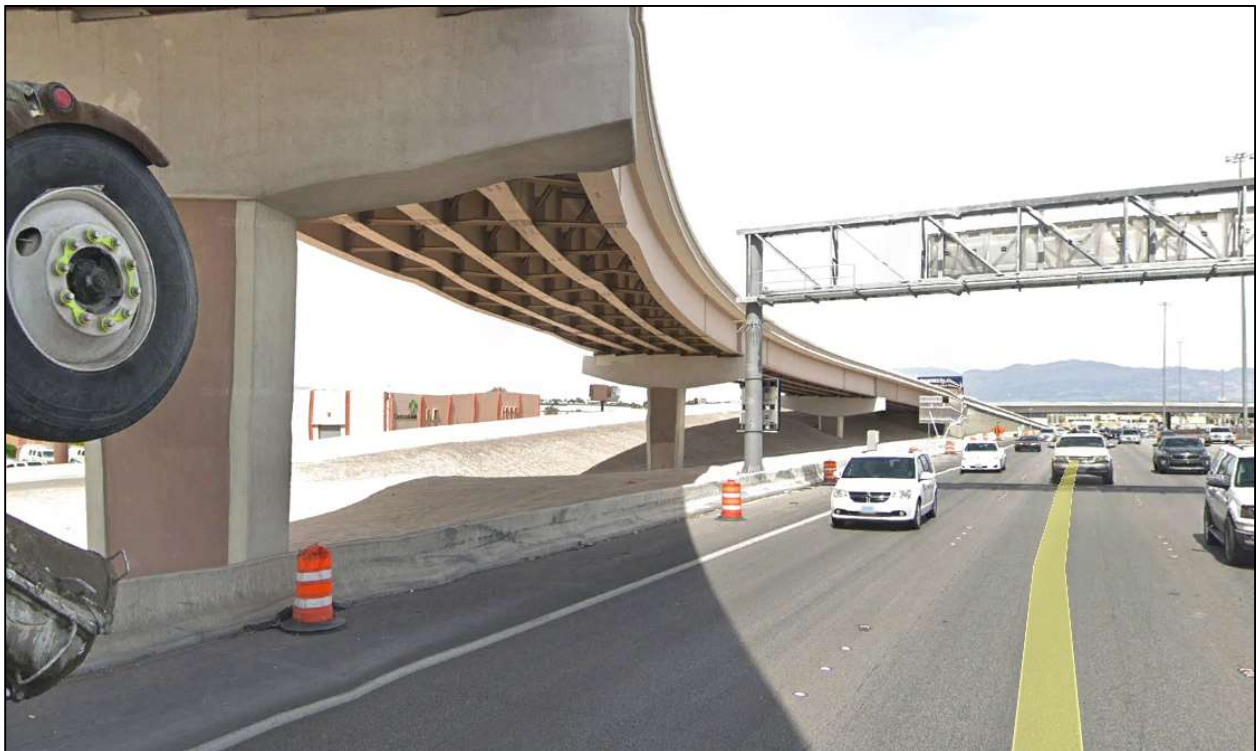
0' to 2' inside and outside shoulders with six 11' lanes (2-11' HOV and 4-11' GP lanes)
