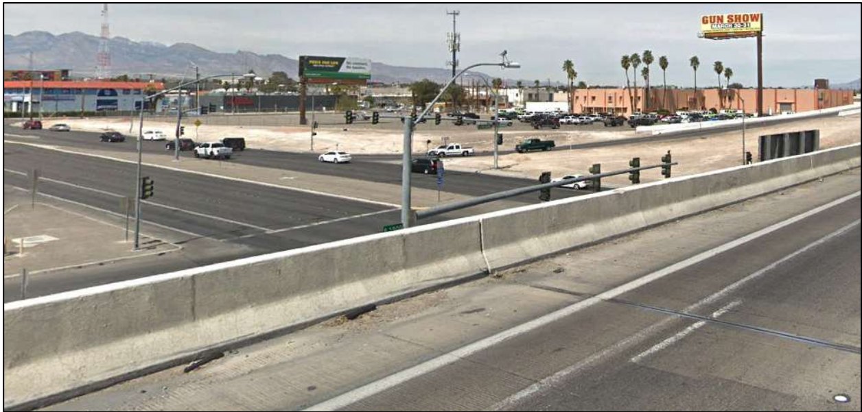
0' to 2' inside and outside shoulder with six 11' lanes (2-11' HOV and 4-11' GP lanes)
