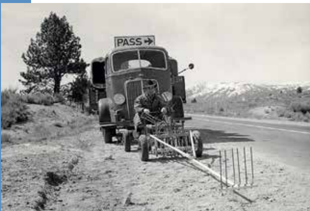
Clear roadway markings save lives
