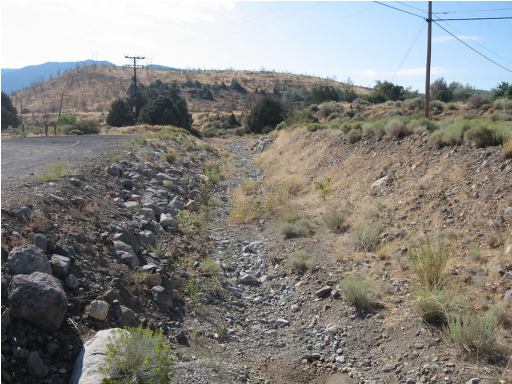
Photo: Bailey Canyon Creek Culvert Crossing at Toll Road. Looking upstream (southeast) at upstream channel. (Photo Date: 9/16/2011)
