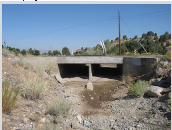
Dual 8'x5' concrete box culverts at Bailey Canyon Creek crossing under Toll Road near Ravazza Road
