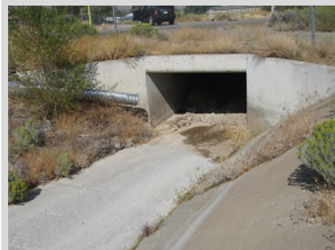
12'x5' concrete box culvert at Bailey Canyon Creek crossing under Kivett Lane
