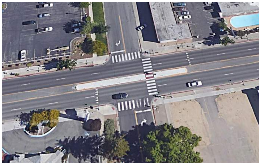
Figure 36: Existing Washington Street Pedestrian Crossing (Source: Google Earth)
