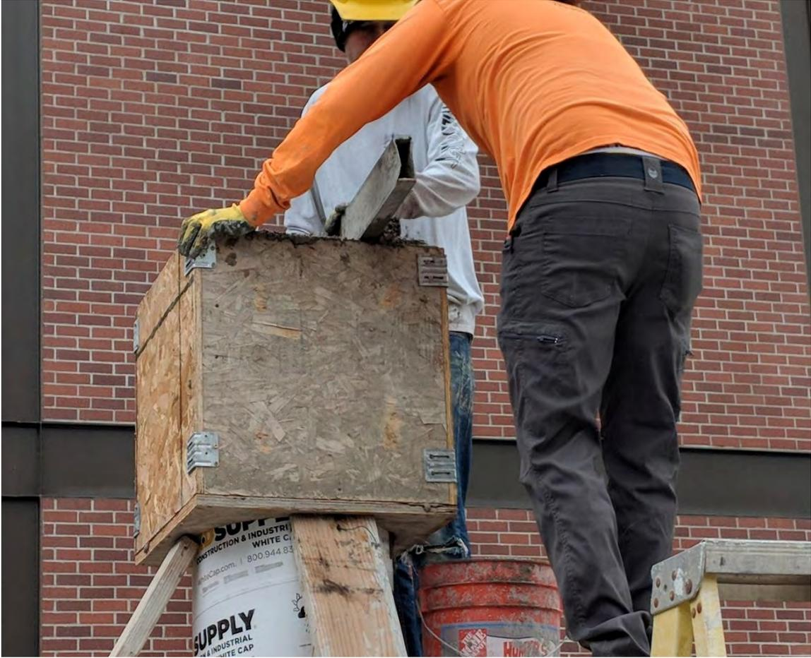
Figure 2.35 Finishing the surface of the loading head
