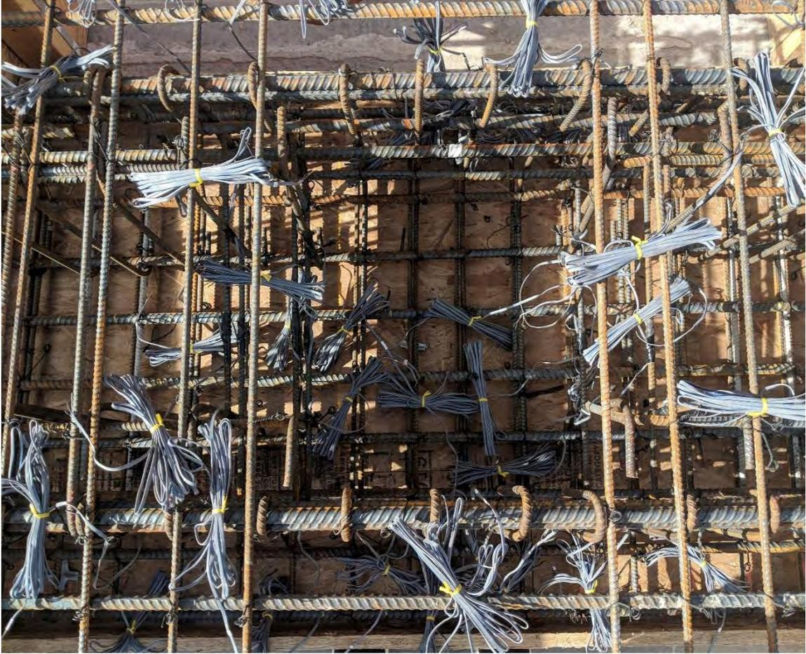
Figure 2.20 Joint reinforcement creating cast-in-place pocket
