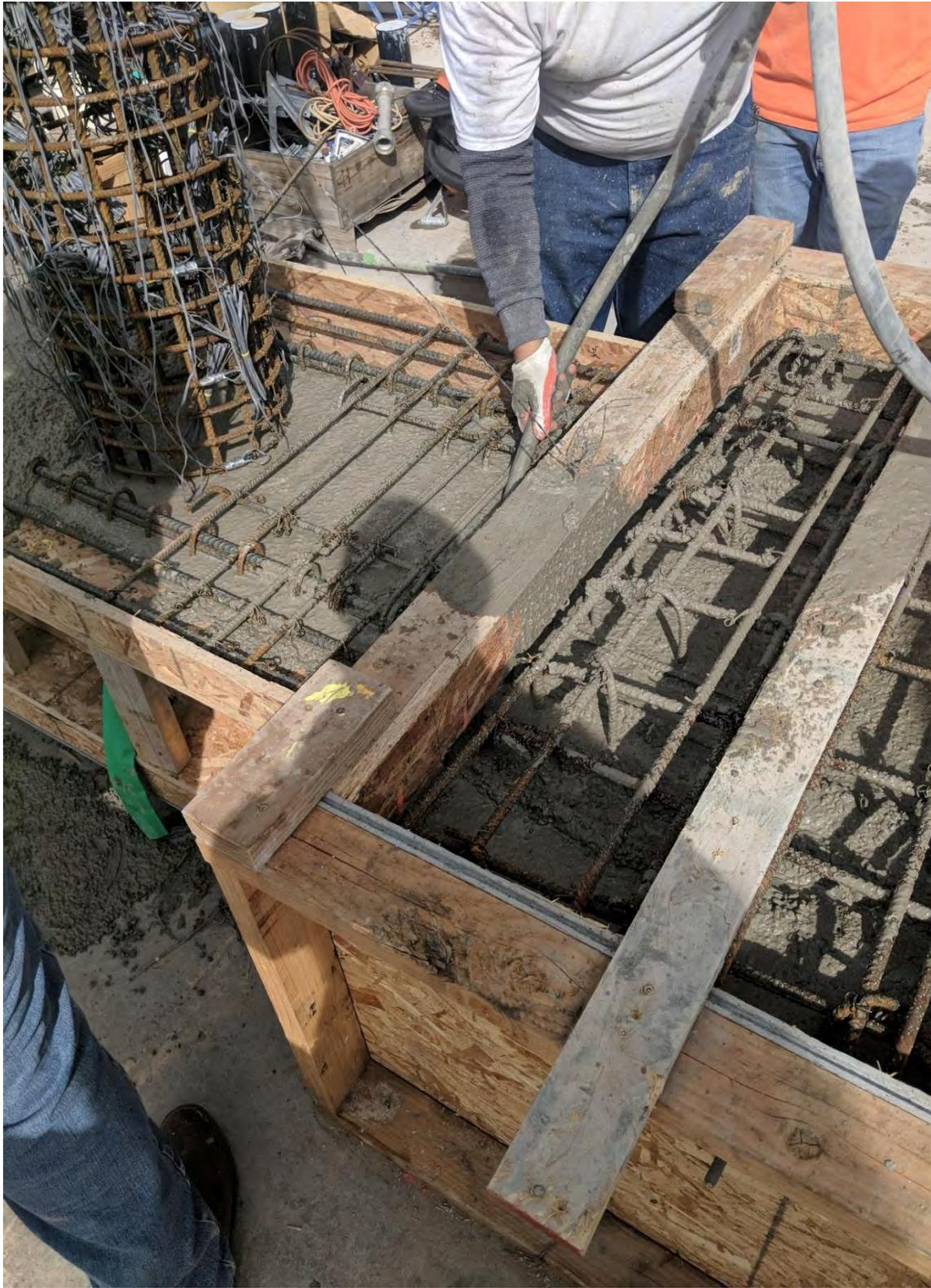
Figure 2.26 Vibrating cap beam concrete
