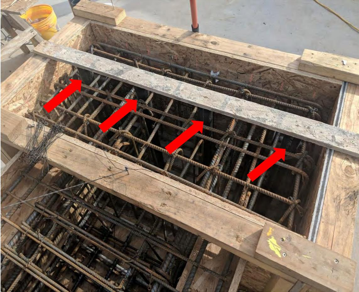
Figure 2.24 PVC pipes placed in an end block
