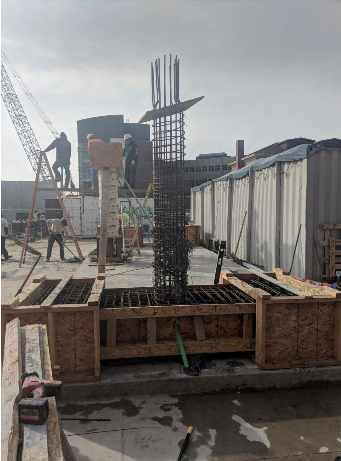
Figure 2.21 Column reinforcement cage placed in pocket
