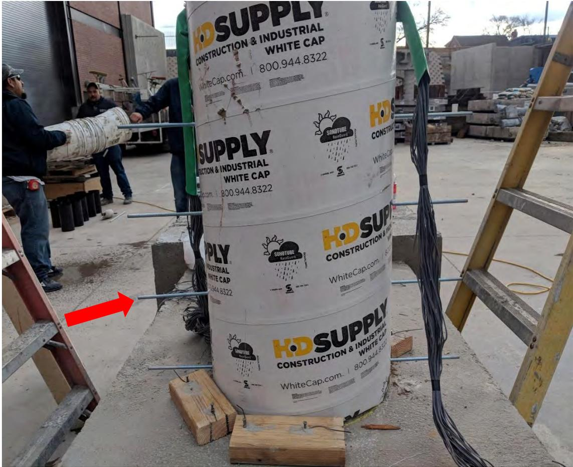
Figure 2.32 Threaded rods for the placement of Novatechniks
