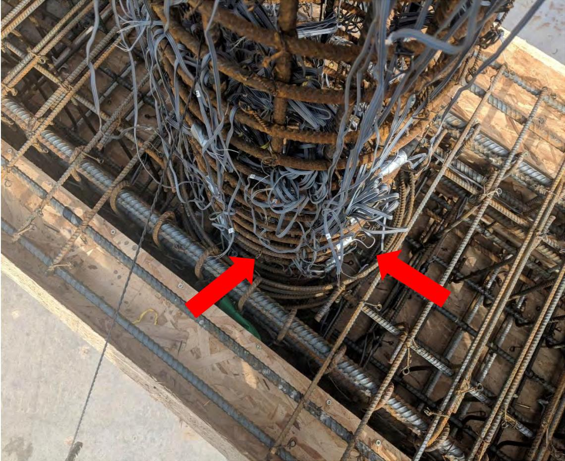
Figure 2.22 Clearance between column reinforcement cage and joint reinforcement
