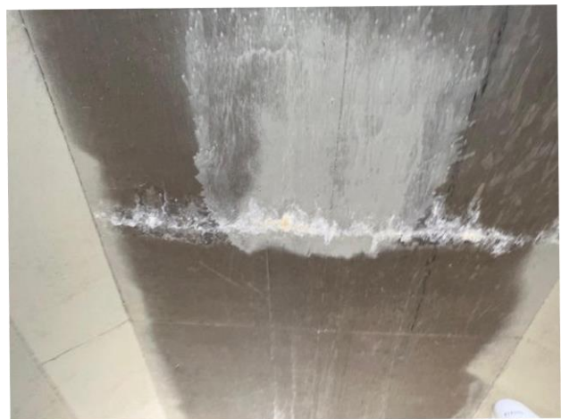
2.2 (4' across the top slab wide view)
