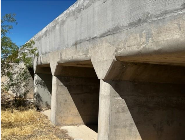
East side of culvert (Construction side)
