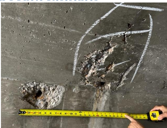
1.2 (8" x 6" drill hole (left) and 18"x12" Spall
