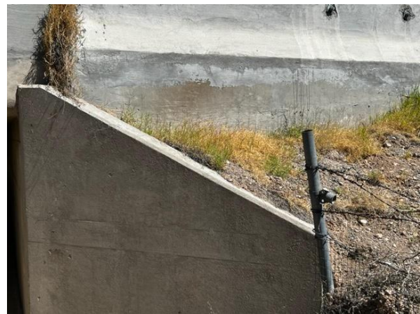
East wing walls (Construction Side)
