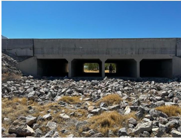
West Elevation (non-construction side)
