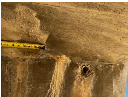
1.5 (shrinkage and exposed bolt)
