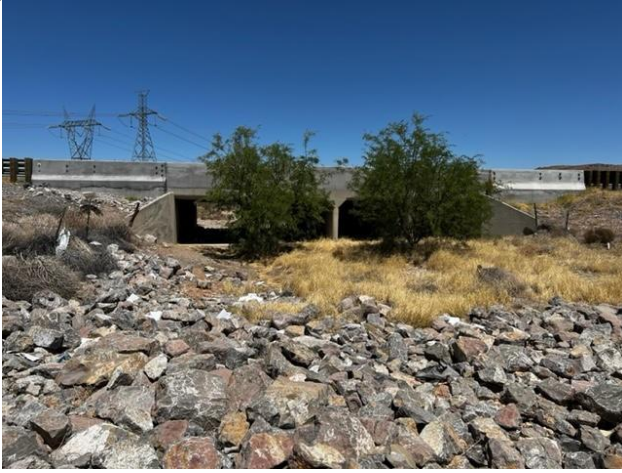
East elevation (Construction side)
