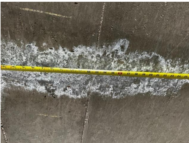
1.3 (26" Efflorescence)
