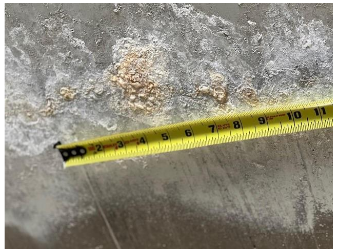
2.2 (4' Efflorescence)
