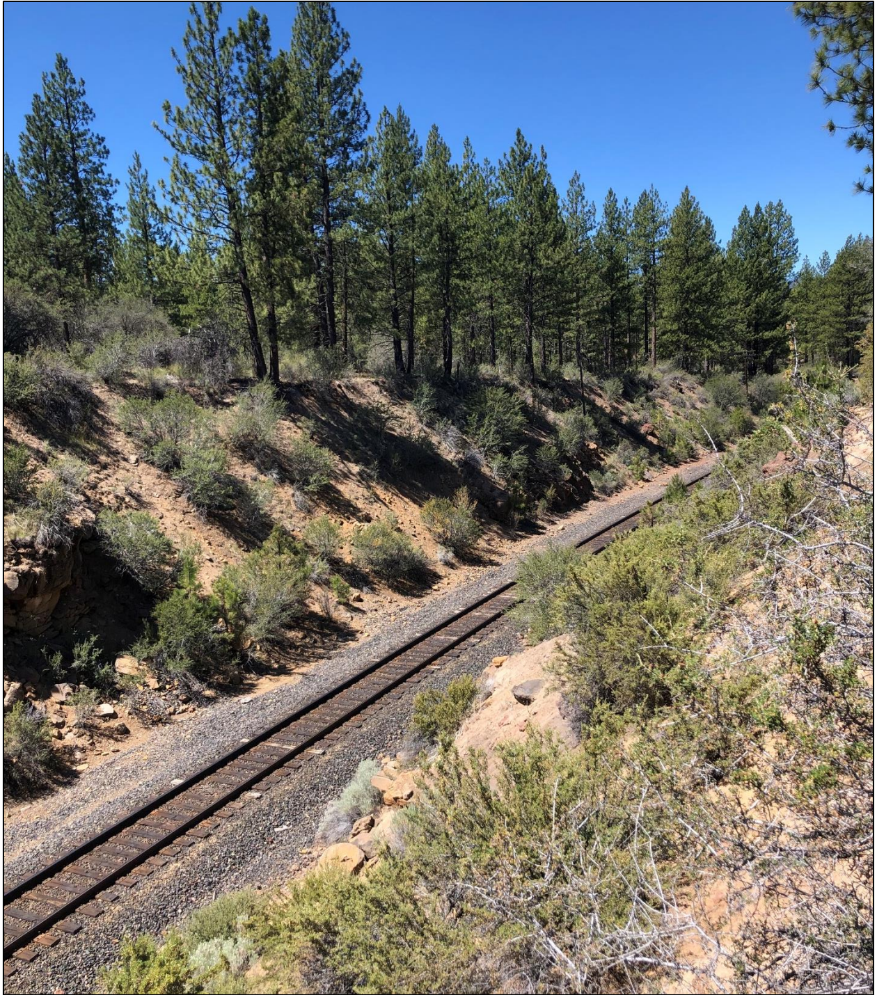
Figure 30: The railroad tracks south of US-97 at Grass Lake B proposed site.
