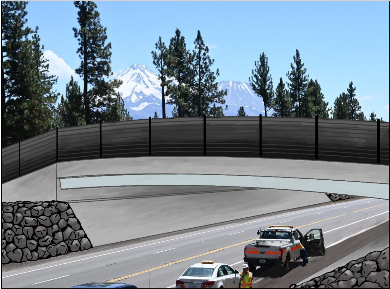
Figure 18: Rendering of US-97 FRP wildlife overpass with Mt. Shasta in the background.
