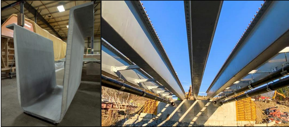
Figure 13: The CT girder bridge system. (a) Left, a cross section of the CT girder showing the foam cores and (b) right, installed CT girders during first construction in Hampden, Maine, 2020.
