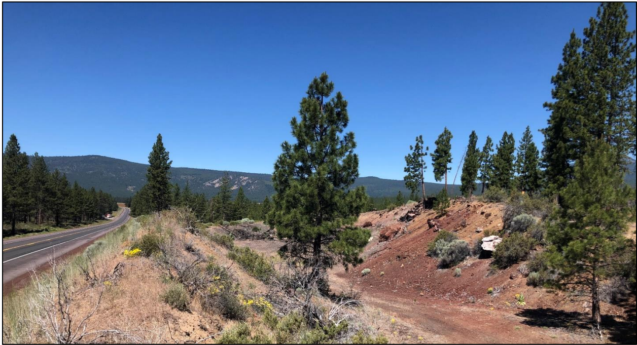
Figure 26: The area north of Grass Lake A potential site that will require backfill to create the approach ramps for the wildlife overpass.
