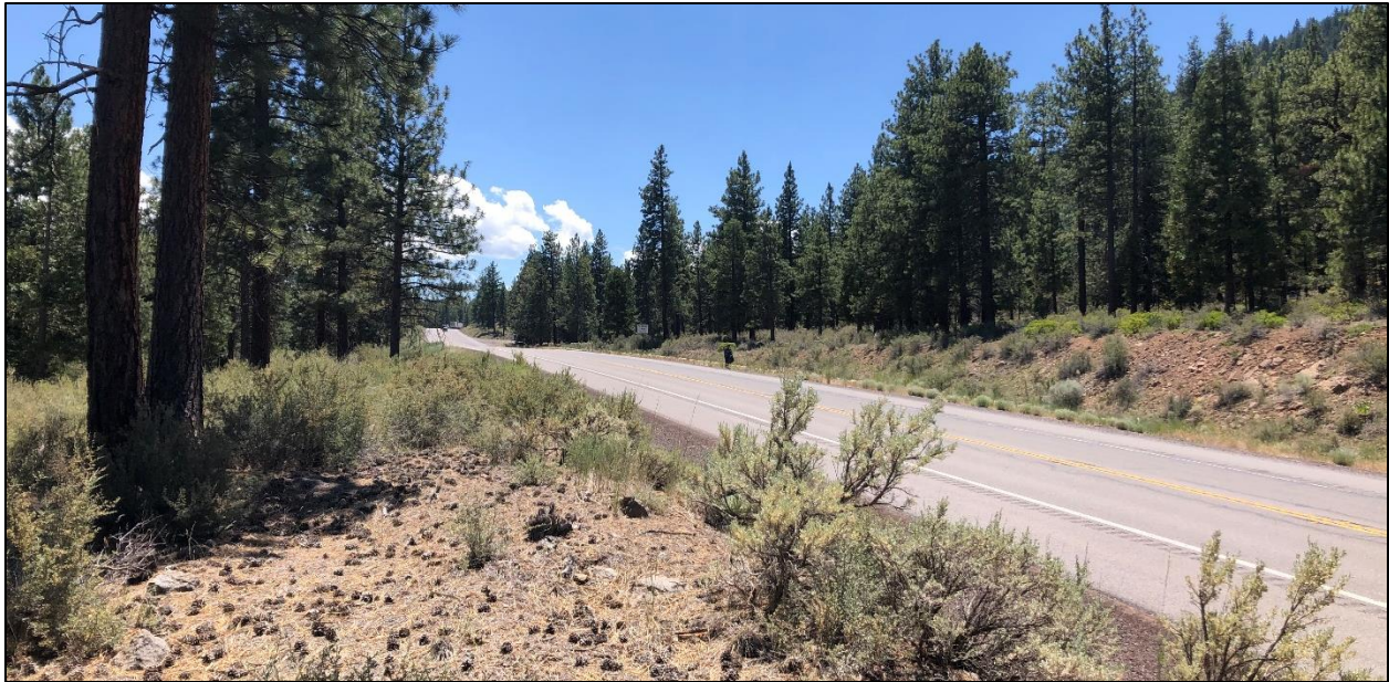
Figure 41: Below grade road alignment at Mud Lake B looking south-southwest.
