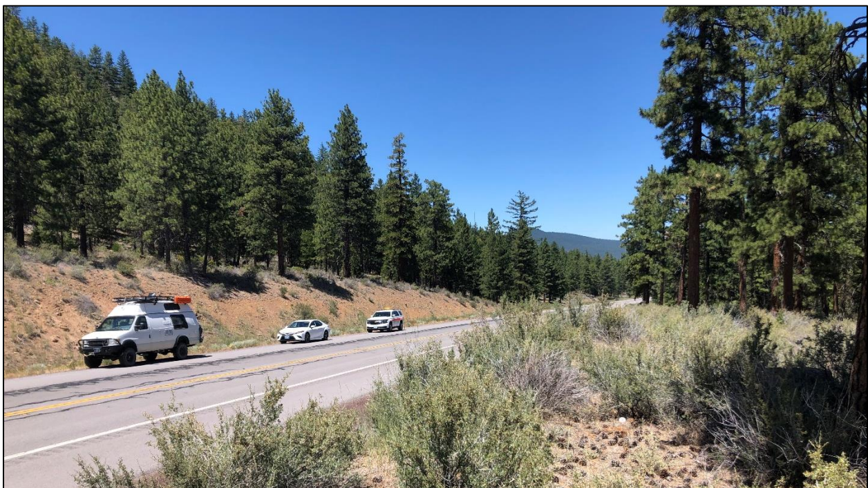
Figure 42: Below grade road alignment at Mud Lake B looking north-northwest.
