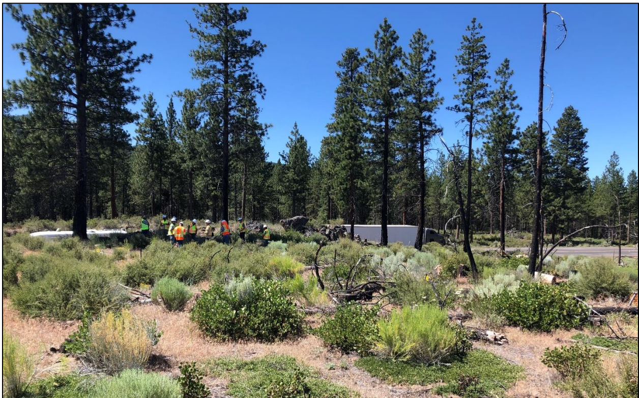
Figure 29: Grass Lake B looking south towards US-97 showing the little fill required for the approach ramps.
