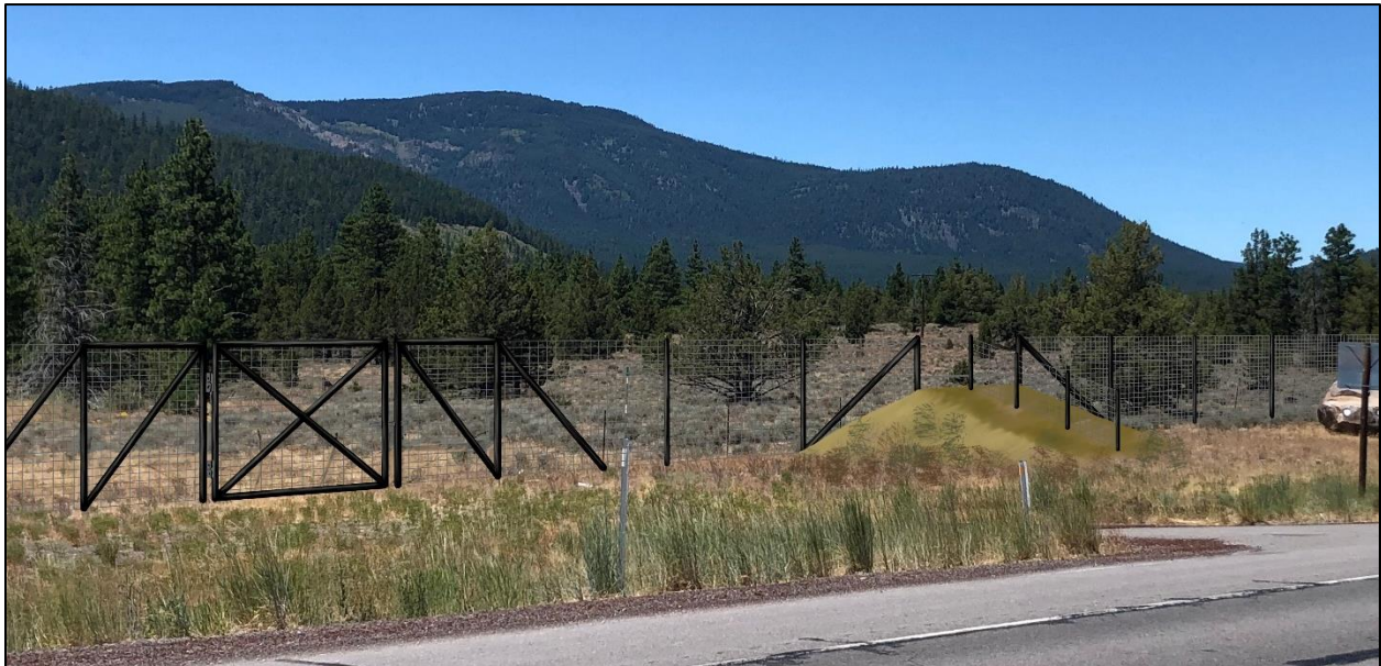
Figure 17: Representation of recycled-plastic posts for use in wildlife fencing, gates, and jump-outs.
