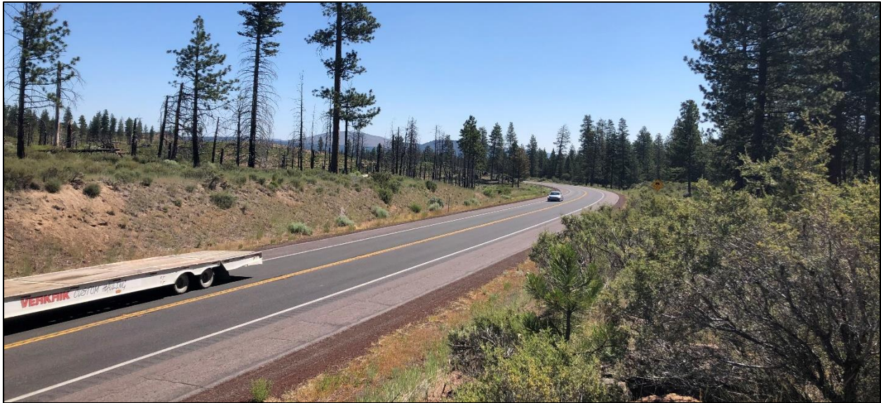
Figure 28: Standing south of US-97 on Grass Lake B looking east-northeast towards the blind curve.
