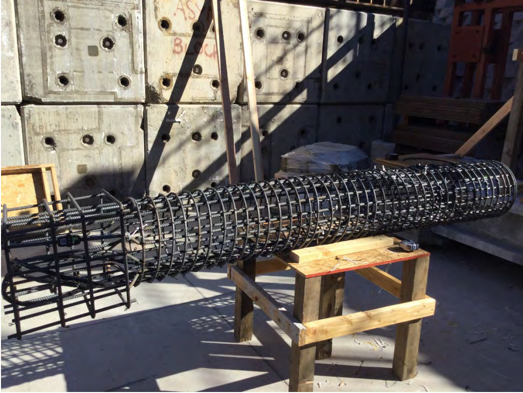
Figure 2.12 Assembled column reinforcement cage and loading head reinforcement
