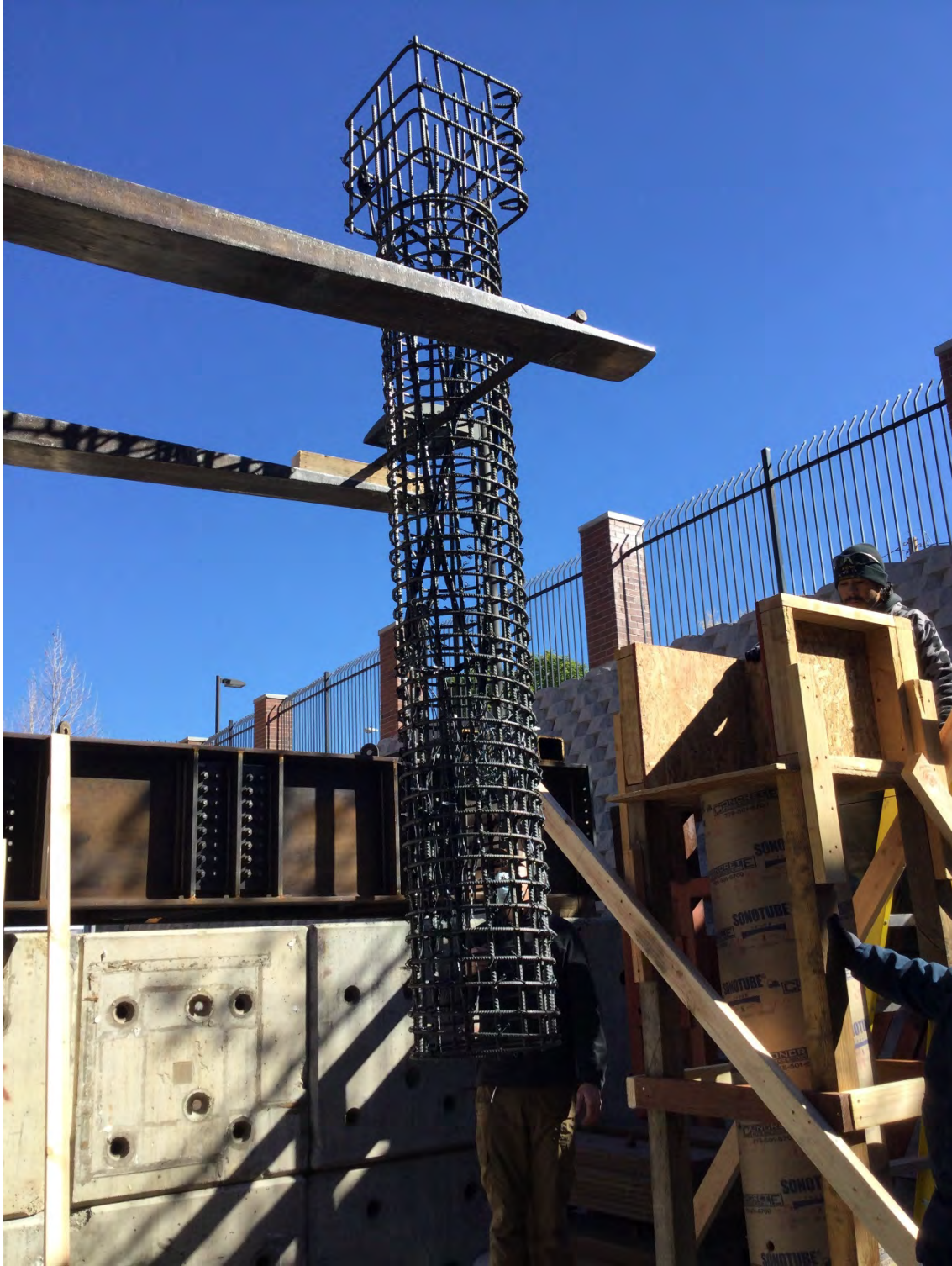
Figure 2.13 Lifting of column reinforcement cage to be placed inside formwork
