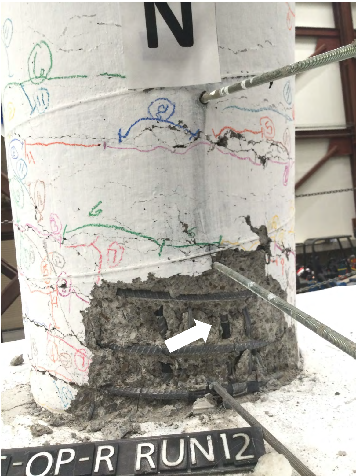
Figure 3.16 Spalling on the north side (run #12)
