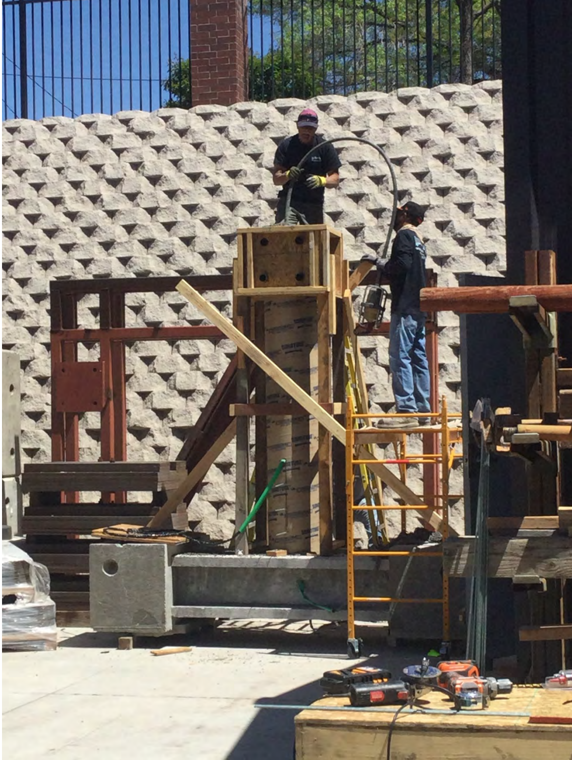
Figure 2.15 Vibrating of fresh cast concrete
