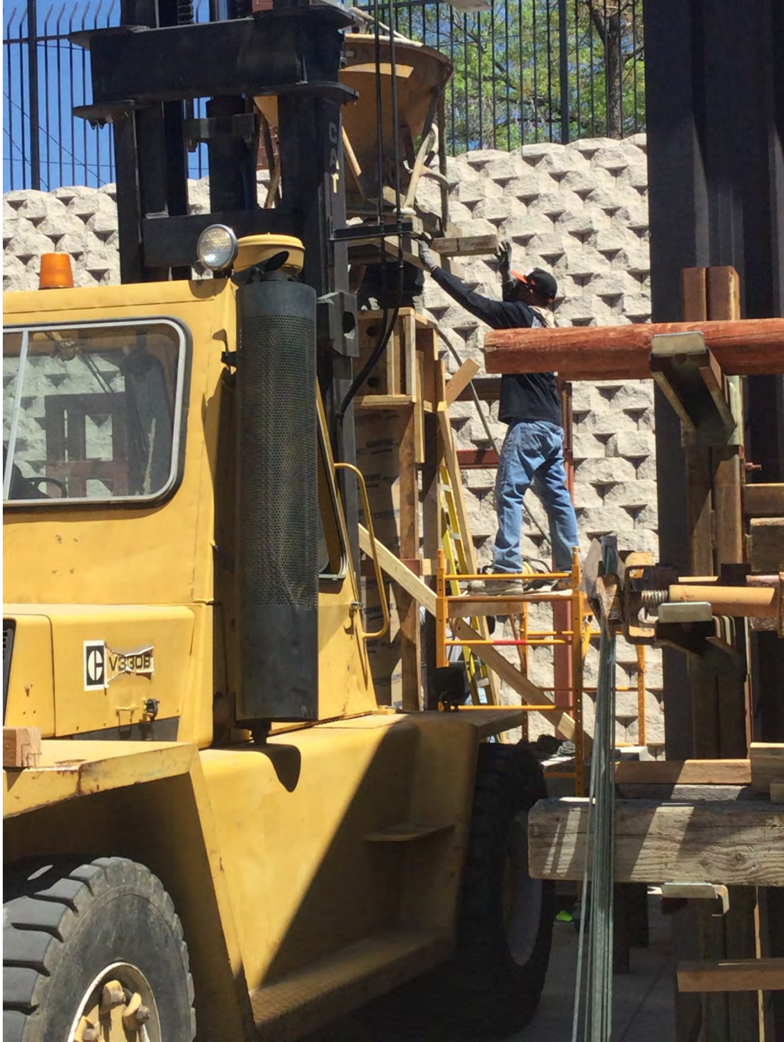
Figure 2.14 Casting of concrete from the top of the column
