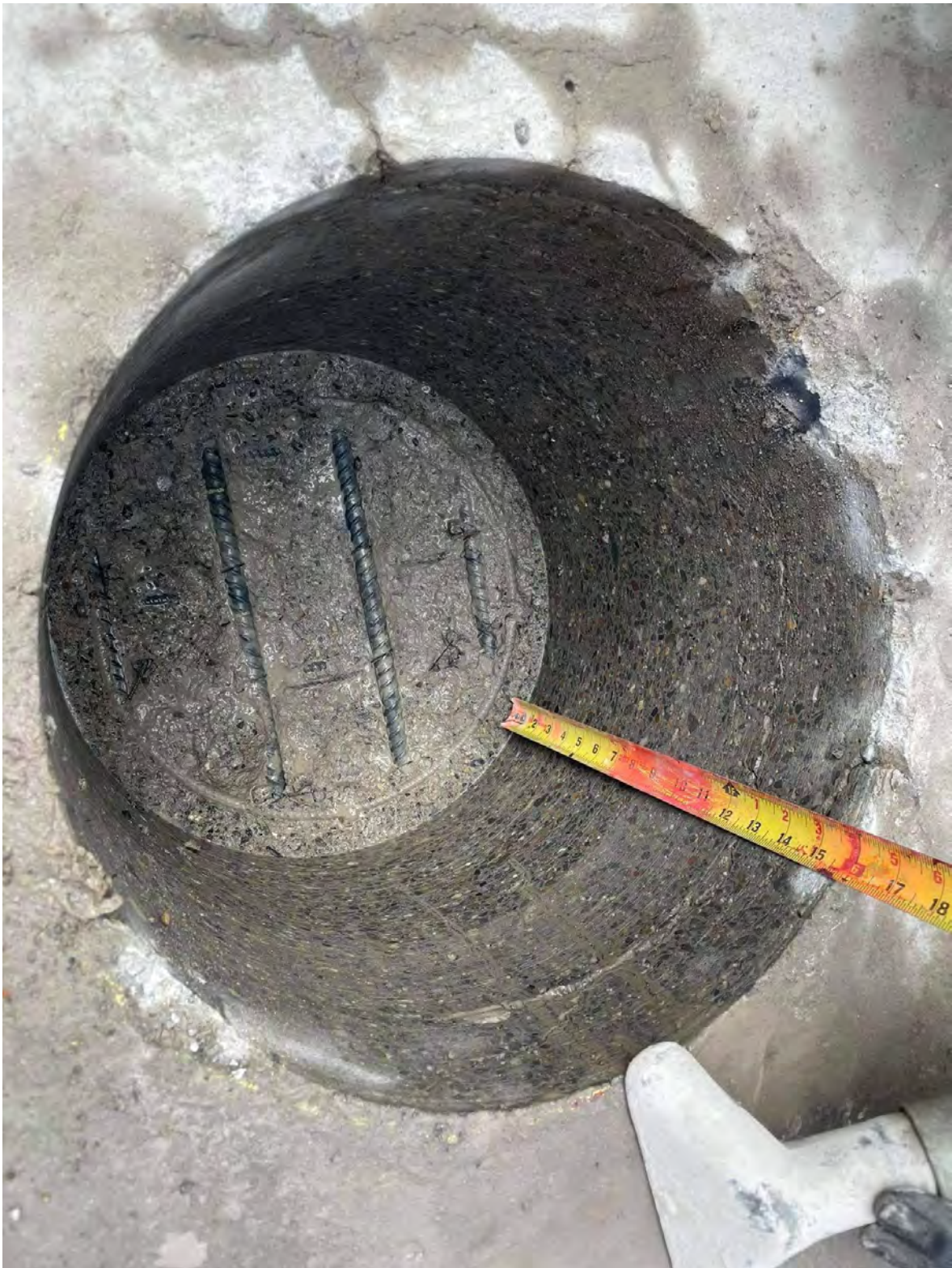
Figure 2.9 Joint pocket after coring
