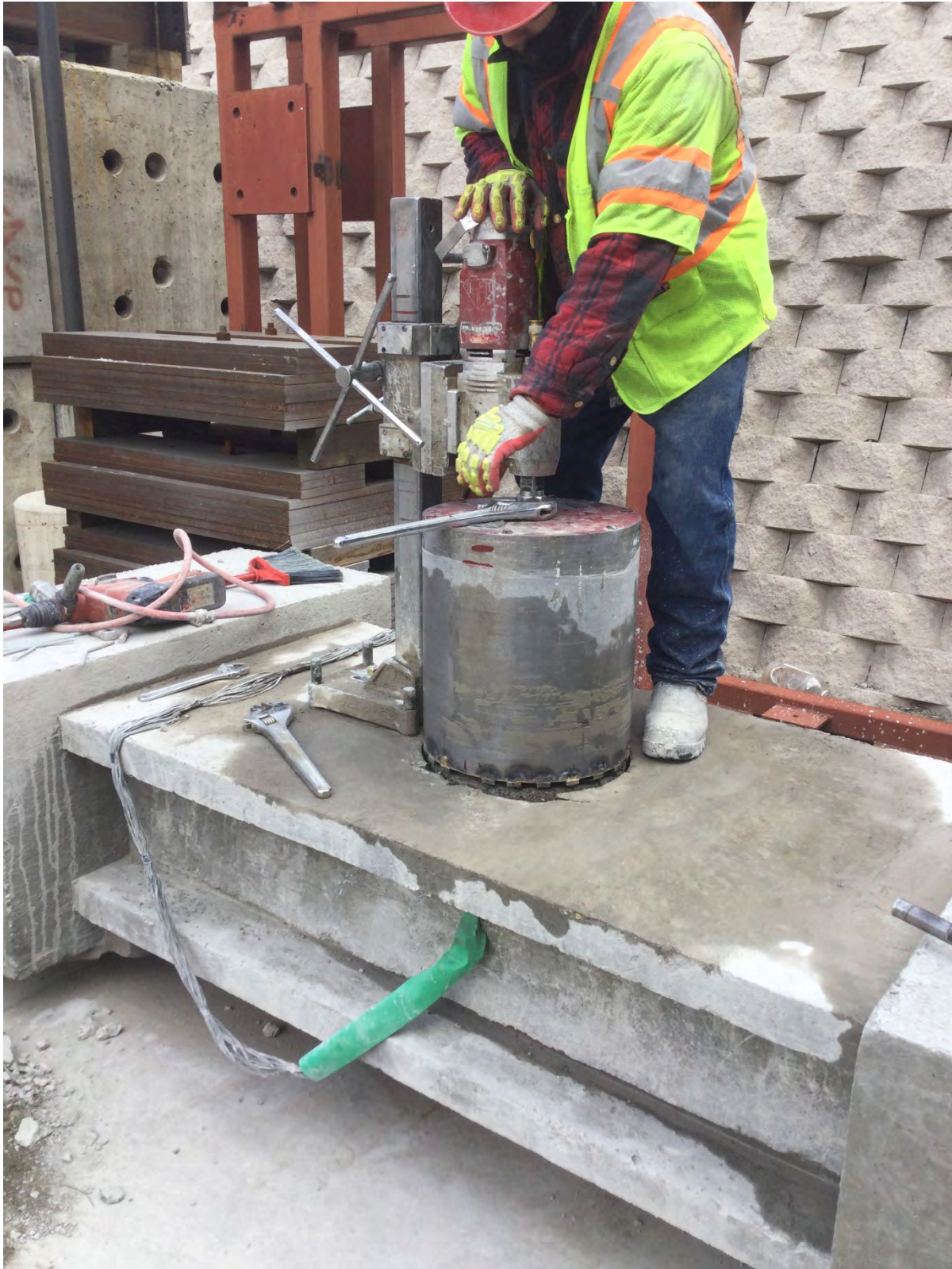
Figure 2.6 Coring process and extraction of older joint
