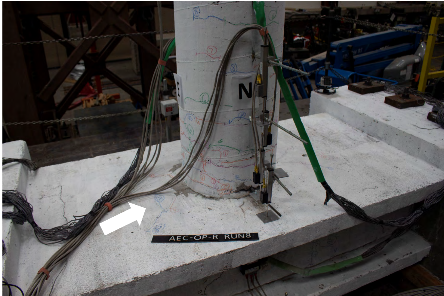
Figure 3.10 Shear crack in the cap beam interface (run #8)
