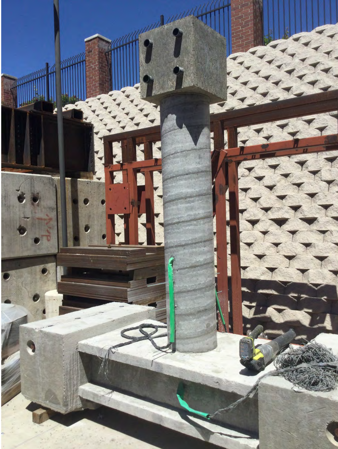
Figure 2.16 Overall specimen after stripping of new column formwork
