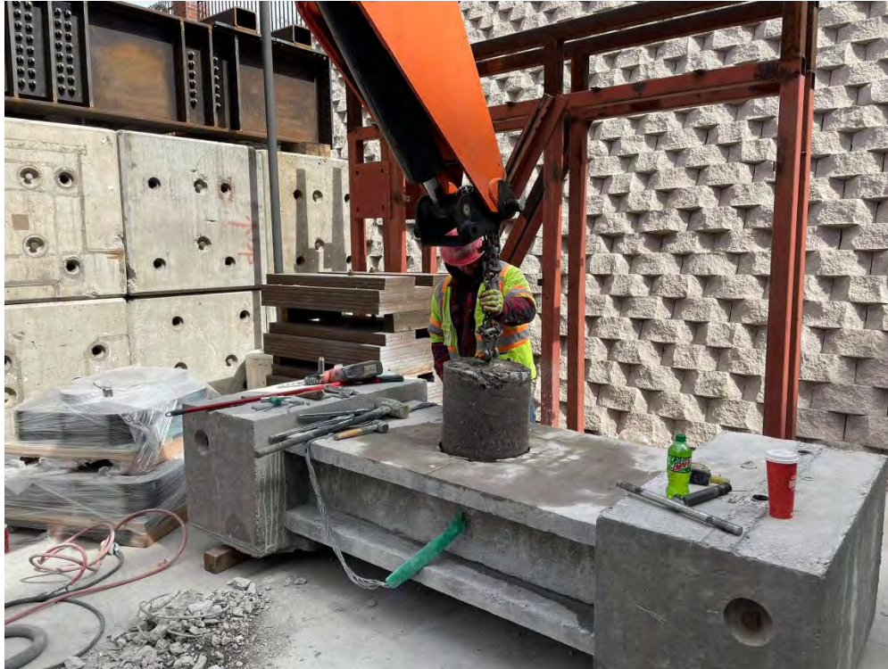
Figure 2.7 Another view of the coring process
