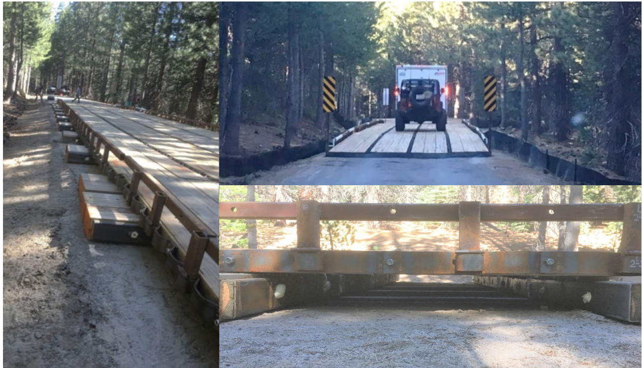
Figure 1. Elevated Road Segment (A) Diagram and (B) Photos; side diagonal view (left), vehicles driving on top of ERS (top-right), side view showing road surface and underneath ERS (bottom-right).
