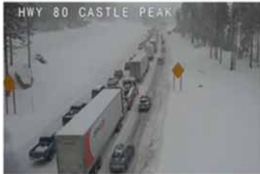
I-80 was closed at the California-Nevada state line on Feb. 22, 2022.
