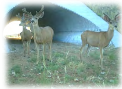
Figure 1. Mule deer exit a wildlife crossing underpass in Utah that was created in a standalone wildlife mitigation project on US 191. Photo Credit: P. Cramer, Utah DOT, & Division of Wildlife Resources.
