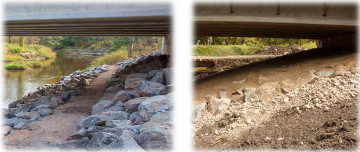
Figure D-4. Minnesota passage bench (left) and aggregate surfacing (right) to treat rip rap to provide soil structure for wildlife and human passage. Photo Credits: Minnesota Department of Natural Resources, courtesy of P. Leete.
