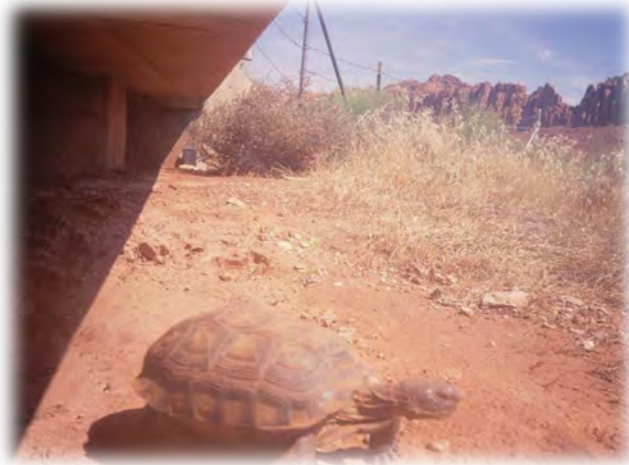
Figure D-18. A desert tortoise moved beneath a wildlife crossing bridge erected less than three feet (1 meter) above the landscape for tortoise passage in St. George, Utah. Photo Credit: A. McLuckie, Utah Division of Wildlife Resources.
