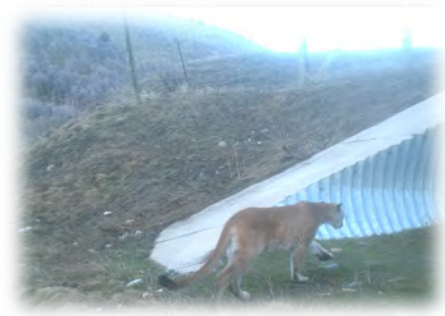
Figure B-9. A mountain lion moves beneath US 89/91 in Utah using a wildlife underpass that was placed when the road was widened from two to four lanes. It was an early wildlife mitigation project in Utah, constructed in 1995. Four wildlife crossing structures were included in the project, which took early planning efforts to integrate into the project. Photo credit: P. Cramer, Utah DOT, Utah Div. of Wildlife Resources, Utah State University.
