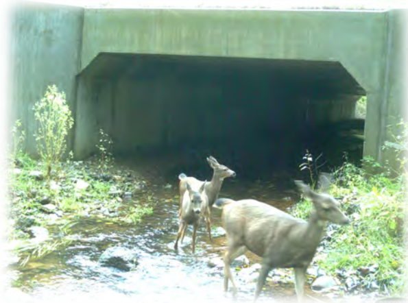
Figure 3-23. Washington DOT fish passage biologists enlarged the size of this fish culvert on US 101 to accommodate terrestrial wildlife for a small cost increase. Photo Credit: P. Cramer, J. Kintsch, and Washington DOT.
