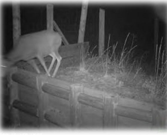
Figure D-37. A Utah high migration escape ramp on US 91. Three sides provide three escape opportunities. Photo Credit: P. Cramer. Photo on Right, Mule deer uses a high migration escape ramp in Utah, US 91. Photo Credit: P. Cramer, Utah DOT, Utah Division of Wildlife Resources.
