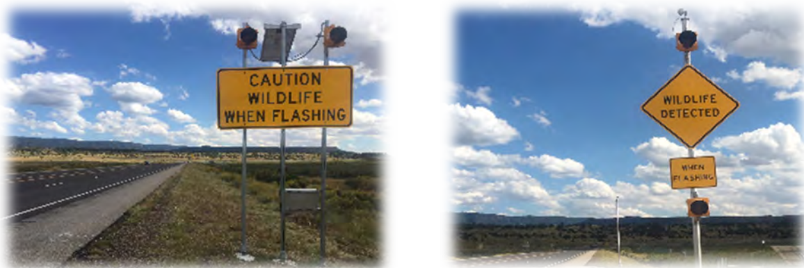
Figure D-59. Wildlife activated driver warning system on US 550, New Mexico. Photo Credit: Arizona Game and Fish Department.
