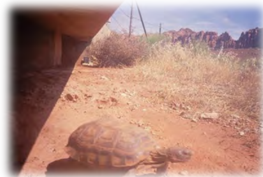
Figure 3-4. Utah DOT and Division of Wildlife Resources worked together to plan for and construct desert tortoise underpasses near St. George, Utah. Photo Credit: A. McLuckie, Utah Division of Wildlife Resources.
