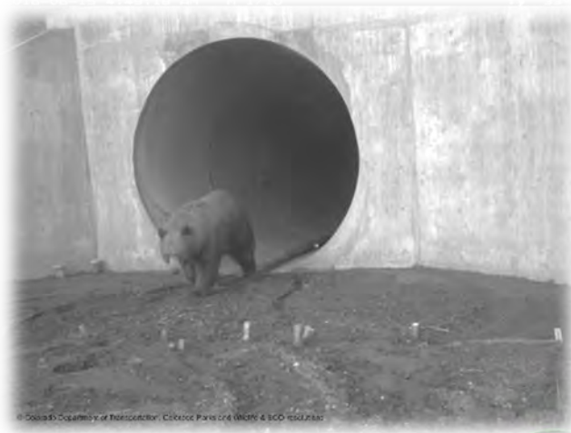
Figure D-27. In Colorado, SR 9, a black bear exits an existing corrugated steel six feet by six feet (2 meters x 2 meters) culvert. Photo Credit: ECO-Resolutions, Colorado Department of Transportation, and Colorado Parks and Wildlife.
