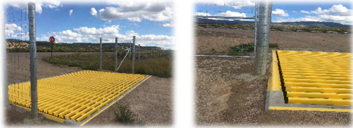
Figure D-45. In New Mexico, along US 550 near Cuba, a double-width cattle guard, (game guard) with perpendicular fence and beveled vault edges to prevent wildlife from walking on them to access fenced right-of-way was placed. Photo Credit: Arizona Game and Fish Department.
