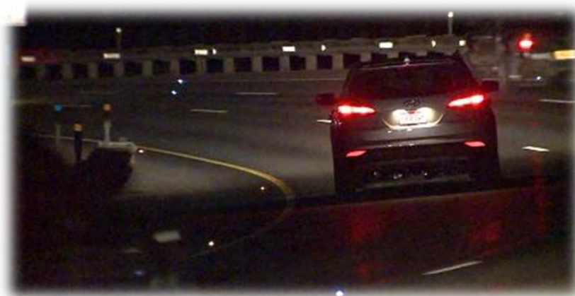
Figure D-61. Solar pucks installed in pavement of Interstate 70 in the mountains outside of Denver. Photo Credit: Fox Denver, KDVR.com.
