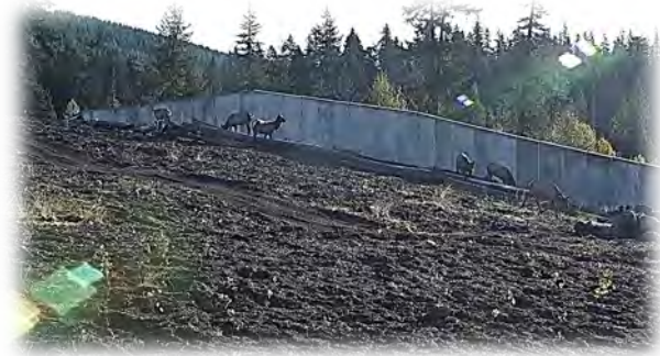
Figure 3-24. Washington DOT constructed a wildlife overpass on Interstate 90, and placed high concrete walls along the sides to shield wildlife from noise and light. The elk that use the structure are comfortable enough there to bed down above the highway. Photo Credit: Washington DOT.
