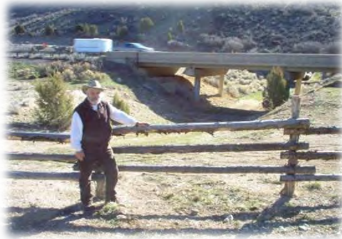
Figure D-29. Utah wildlife rail fence at a wildlife crossing structure under Interstate 15. The intent was to keep out livestock but allow wildlife access. Photo Credit: P. Cramer.
