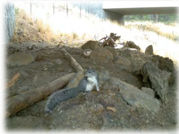
Figure D-5. Oregon's US 97 Lave Butte Wildlife Mitigation Project placed stumps, logs, and rock along a wildlife underpass set of bridges for small animal movement. Photo Credit: Oregon Department of Transportation, Portland State University, P. Cramer.
