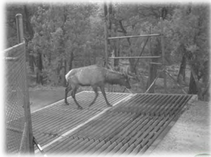
Figure D-41. Elk breached double cattle guard in Arizona. Photo Credit: Arizona Game and Fish Department and Arizona DOT.
