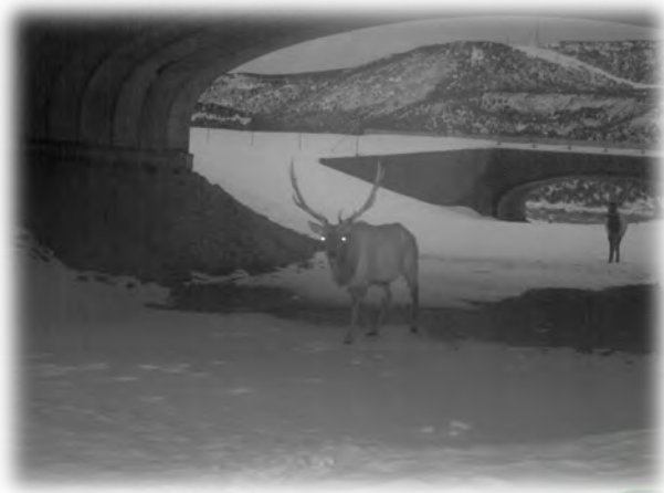
Figure 3-29. Bull elk moved beneath Interstate 70 through pre-fabricated arch wildlife underpasses in Utah. However, only several female elk were compelled to do so, even with the arch widths of 60 feet (18 meters). Photo Credit: P. Cramer, Utah DOT, Utah Division of Wildlife Resources.
