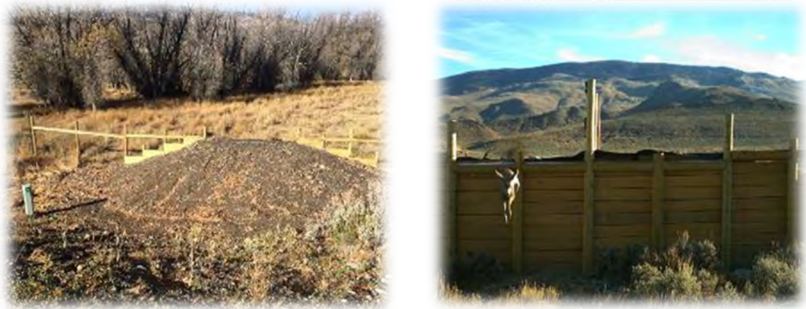
Figure D-35. Left, Colorado SH 9 most successful escape ramp type with a 3:1 slope and no center fence. Photo Credit: P. Cramer. Right, mule deer used an escape ramp with center fence in Colorado, SR 9. Photo Credit: Colorado DOT, Colorado Parks and Wildlife, ECO-resolutions.
