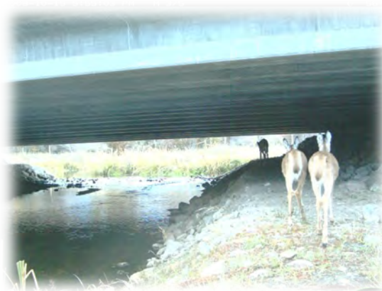
Figure 3-30. White-tailed deer moved beneath bridges less than five feet (1.5 meters) in height under US 93 in Montana. Photo Credit: P. Cramer, Montana DOT.
