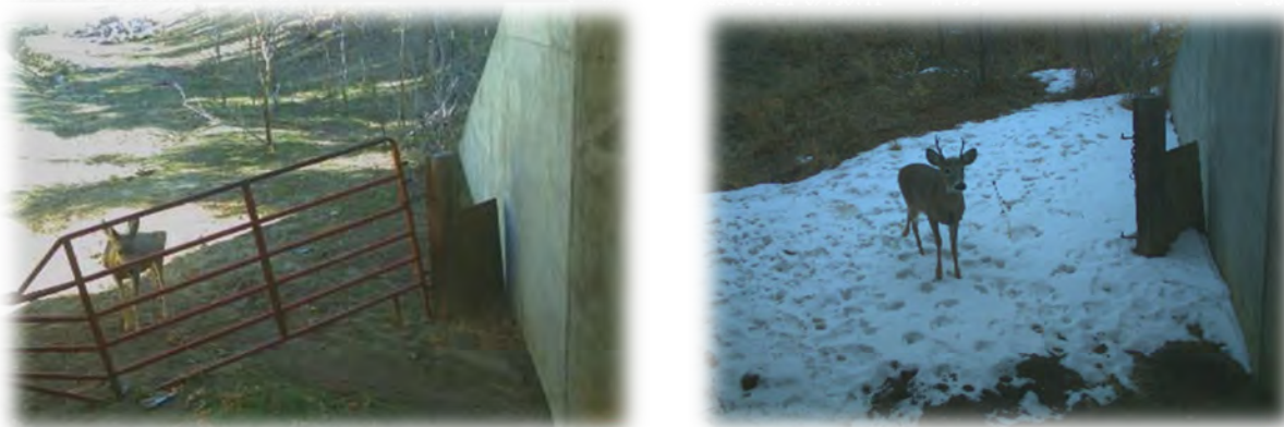
Figure D-6. In New Mexico, a gate located at a culvert prevented nearby livestock and wildlife from moving beneath the road, (left). When the gate was removed and a right-of-way fence installed 40-feet (12 meters) from the culvert entrance, mule deer began moving through, with over 880 mule deer successful crossings, (right). Photo Credit: Arizona Game and Fish Department and New Mexico Department of Transportation.
