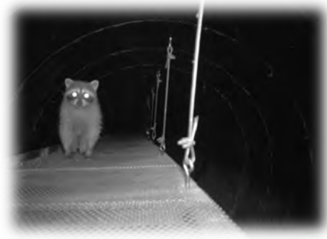
Figure 2-3. Raccoon used a shelf placed in an existing culvert to pass beneath US 93 in Montana. Photo Credit: P. Cramer and Montana DOT.
