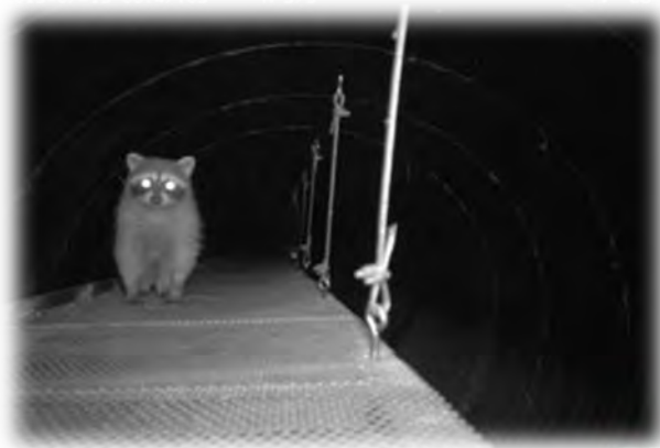
Figure D-2. A small mammal shelf was placed in a Montana US 93 culvert to facilitate movement of raccoons and other wildlife. Photo Credit: P. Cramer and Montana Department of Transportation.
