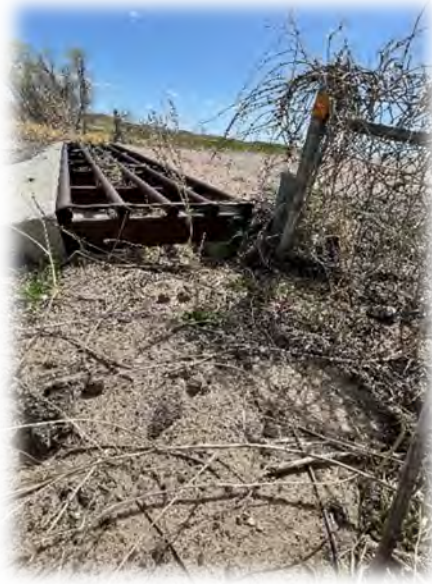
Figure D-46. A small animal guard along a turtle fence on Valentine National Refuge in Nebraska allowed turtles and others to fall back to ground level and to try to move along the fence rather than cross over the road. Note painted turtle along the fence. Photo Credit: P. Cramer.
