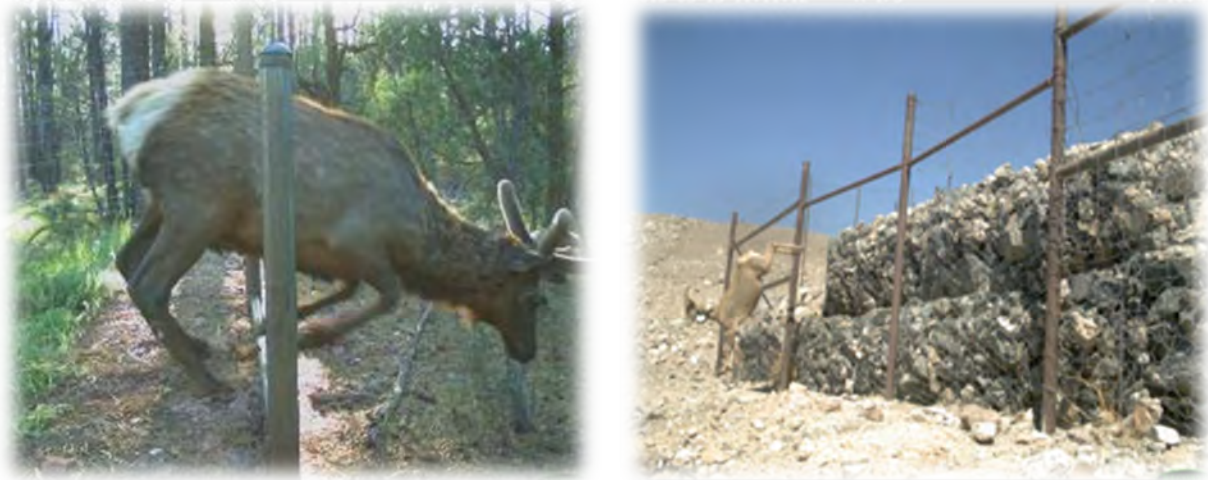
Figure D-38. Left, elk used escape ramp and right, desert bighorn sheep used a six feet (1.8 meter) high escape ramp, both in Arizona. The bar on the desert bighorn ramp was placed higher than six feet (1.8 meter). Photo Credit: Arizona Game and Fish and Arizona DOT.
