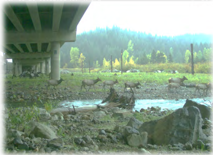
Figure 4-13. Elk use the Gold Creek Bridge beneath Interstate 90 in Washington. This was one of over one dozen wildlife crossing structures built in this section of Interstate 90. Photo Credit: Washington DOT.
