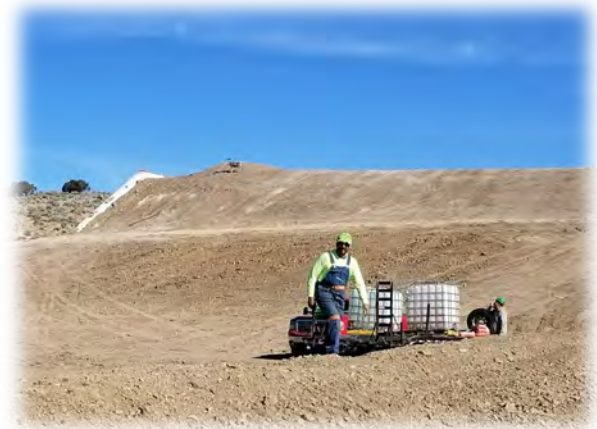
Figure 3-35. The wildlife overpasses constructed over Interstate 80 in Nevada were so well placed and designed, a mule deer couldn't wait until construction was over to use the overpass during the last phase of construction. Photo Credit: Unknown Construction Personnel.
