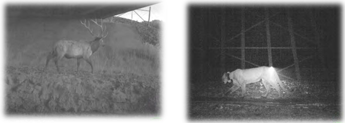
Figure D-17. In New Mexico, left, elk moved beneath the US 550 bridge near Cuba, and right, in Tijeras Canyon mountain lion walked below the bridge under Interstate 40. Photo Credit: Arizona Game and Fish Department and New Mexico Department of Transportation.
