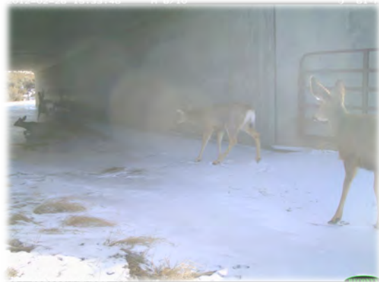
Figure 3-41. Maintaining wildlife crossing culverts and other culverts used by wildlife to keep them free of ice buildup is a maintenance task that may be a new responsibility. Here mule deer fell on ice in a culvert. Photo Credit: P. Cramer, M. Schwender, and Idaho Game and Fish.
