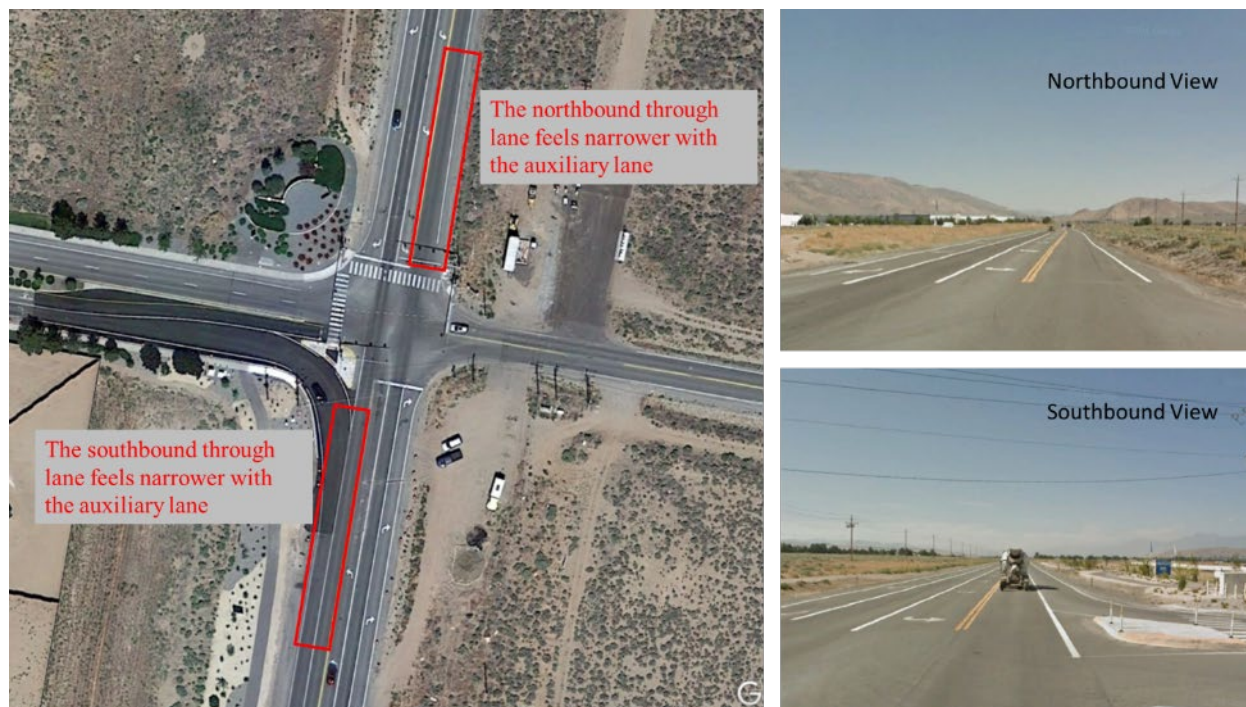
Figure 8-8 Comparison of northbound and southbound geometric elements that may have helped to reduce the southbound traffic speeds
