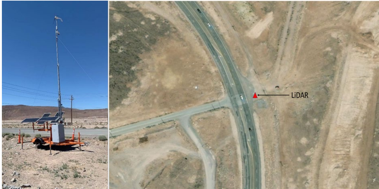
Figure 12-3 Trailer for data collection(left) and Top view of the site and the location of the LiDAR (Right)
