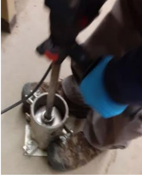
Figure 4.21. Compaction with vibratory compactor.
