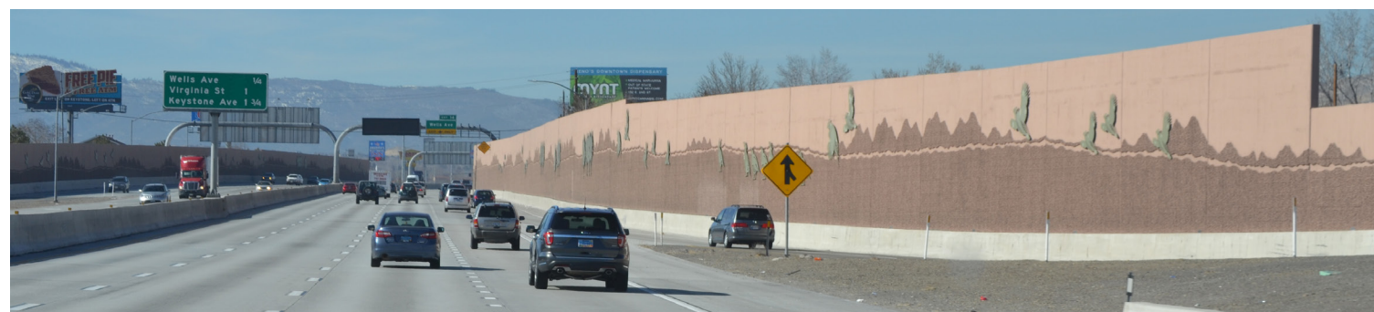
This existing traffic noise barrier at the I-80/Wells Avenue interchange includes an artistic treatment. Traffic noise barriers are practical, reasonable, and effective for minimizing and mitigating noise impacts.
