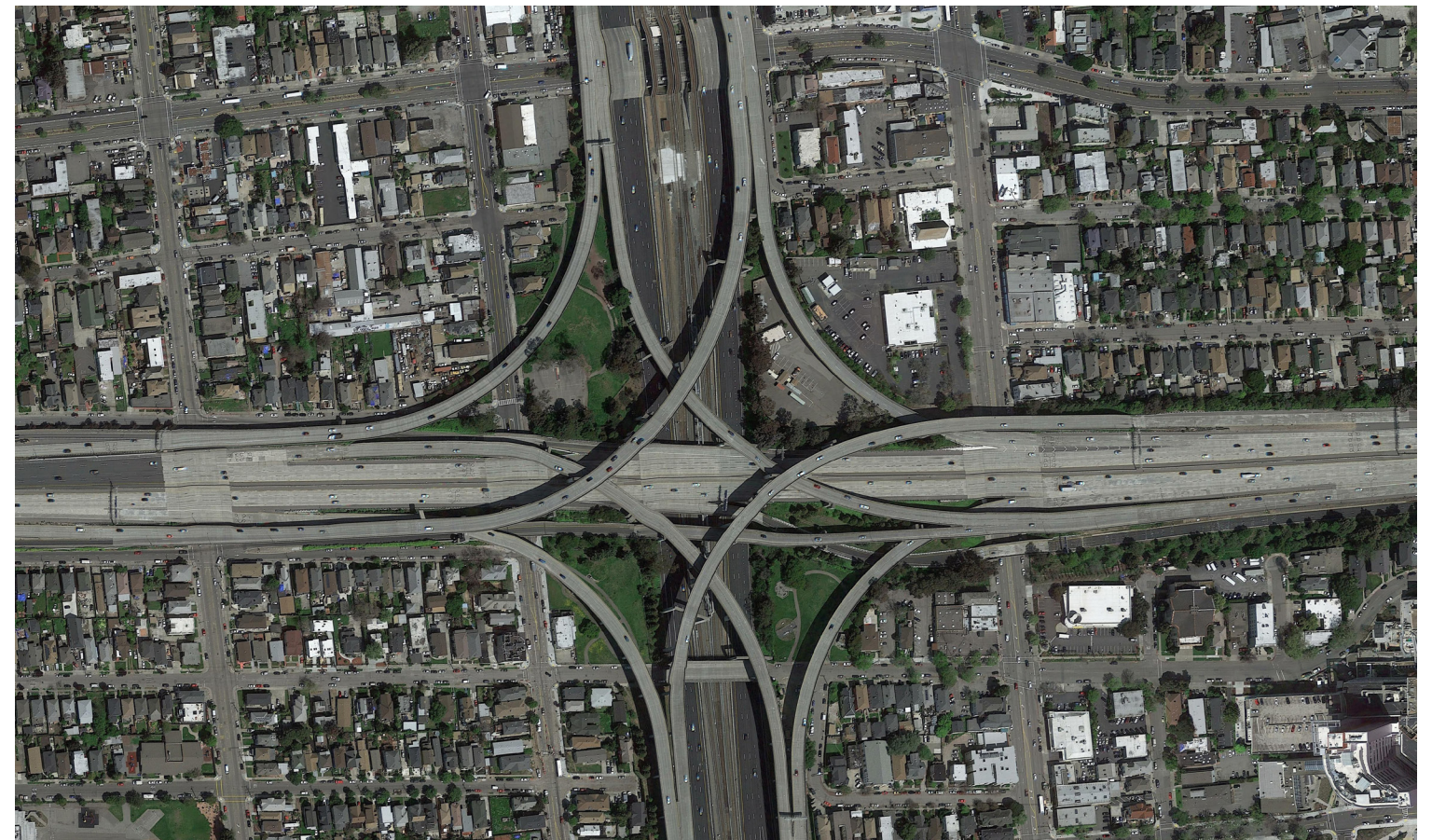
SR-124 and I-580 Interchange in Oakland, California. © 2019 Google
