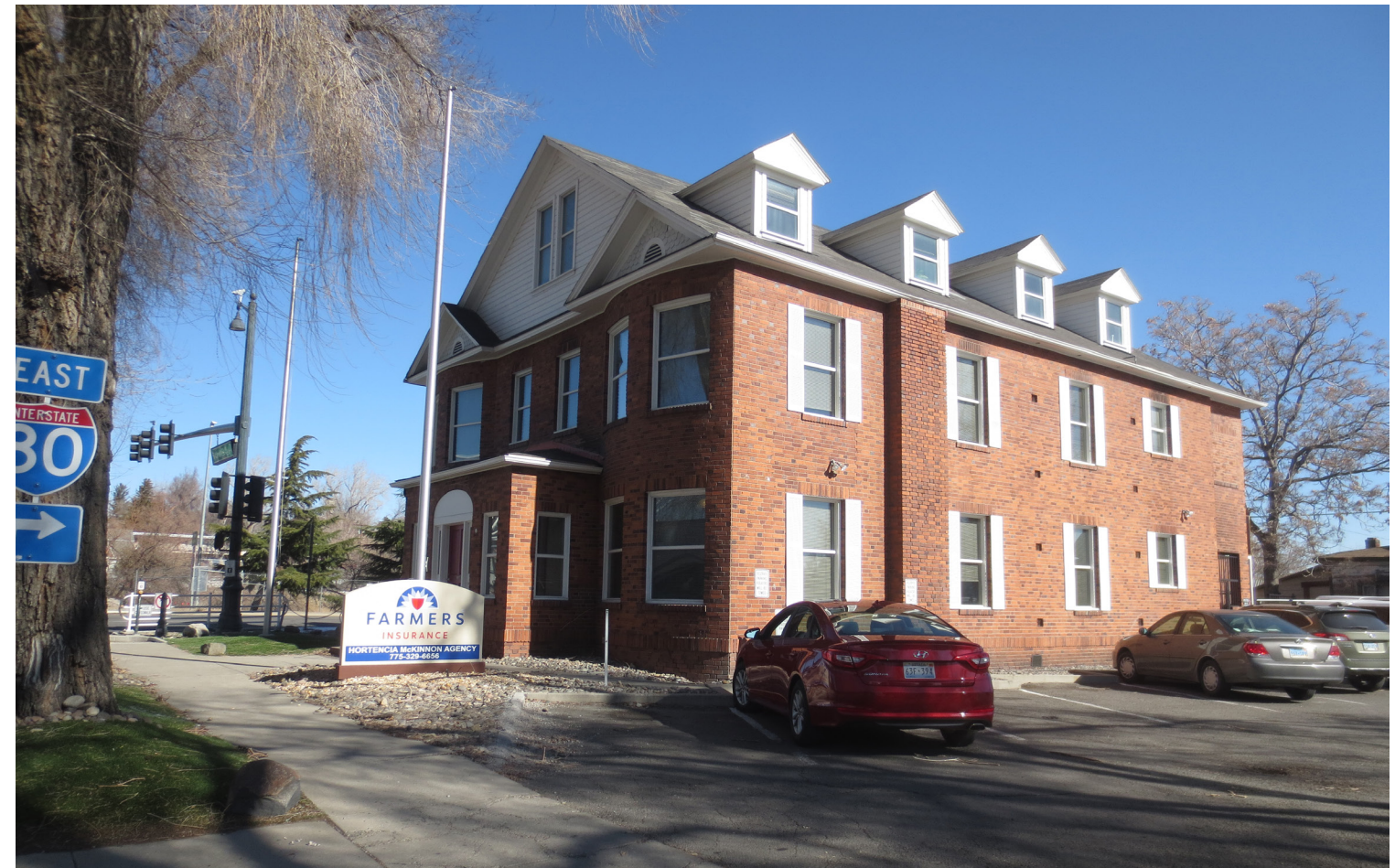
Francovich Office Building
