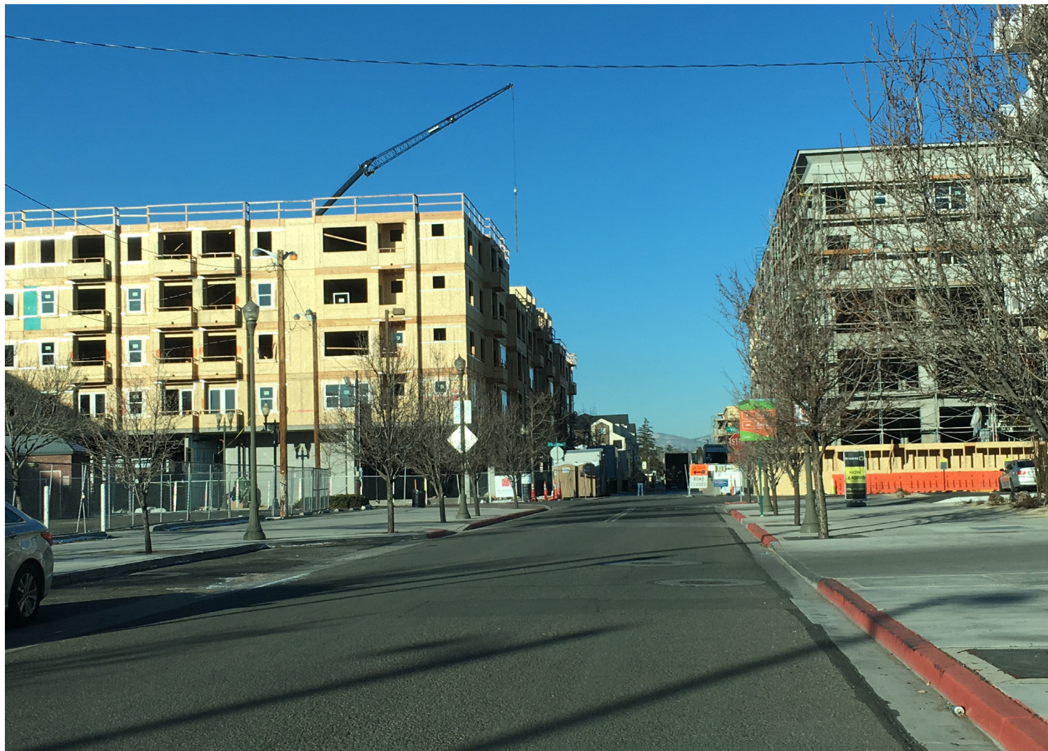
Apartment construction in Sparks
