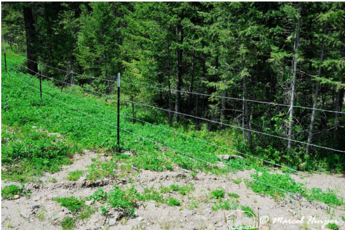
Figure 59. Wildlife friendly livestock fence with smooth top and bottom wires, Montana, USA.
