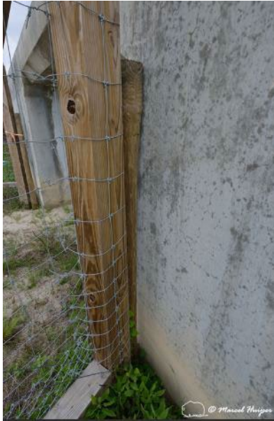
Figure 52. Tight connection (no gap) between last fence post and wall of the wildlife underpass, Hwy 331, Hwy 83 near Freeport, Florida, USA. The angle at which the fence comes in does not result in a dangerous wedge or funnel that could lead to animals getting trapped.
