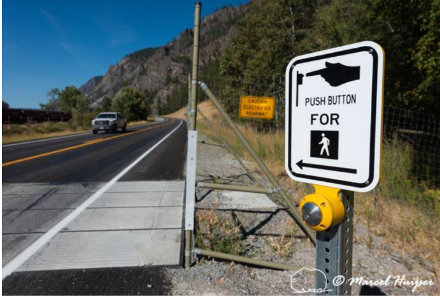
Figure 40. Push button on timer (turns electricity off for 1 minute) for pedestrians at an electrified barrier embedded in travel lanes to keep large mammals, including bighorn sheep, out of fenced road corridor, MT Hwy 200, Thompson Falls, Montana, USA.
