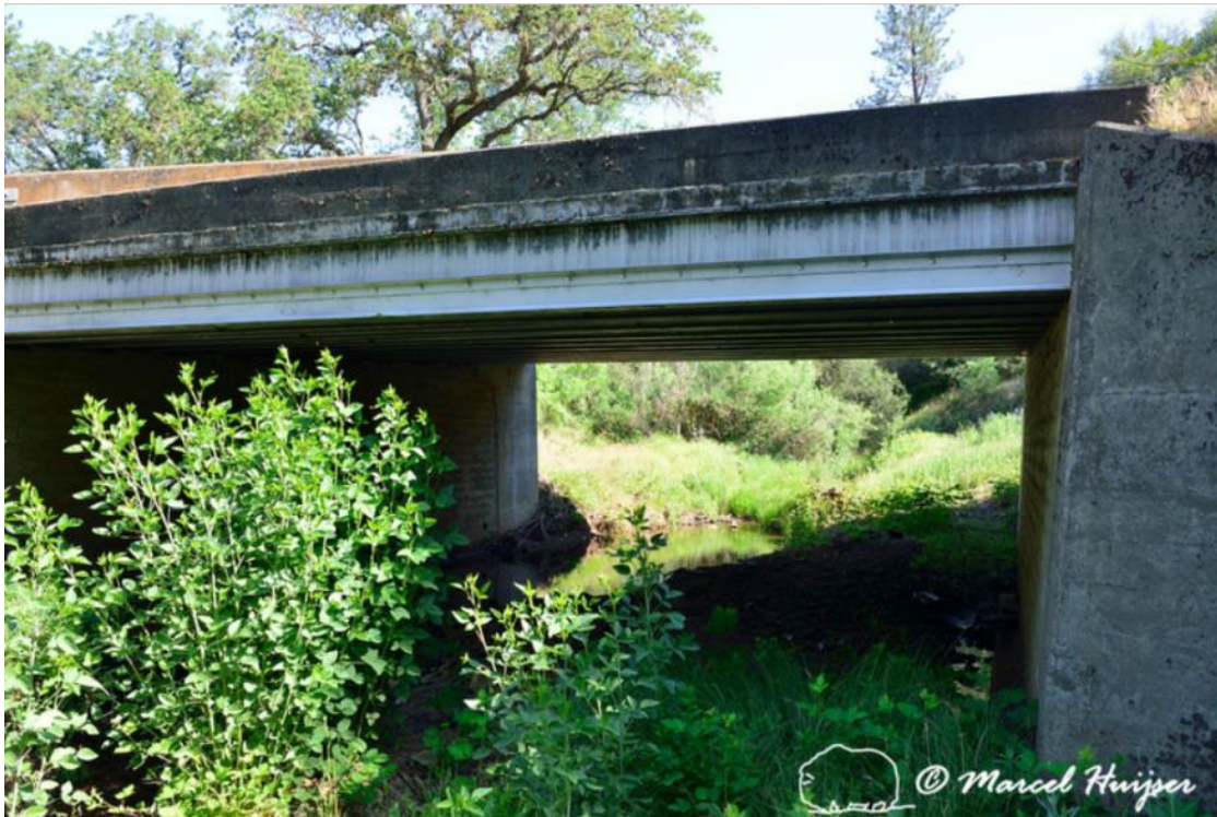
Figure 24. Bottomless multifunctional underpass, Hwy 88 near Jackson, California, USA. The underpass is for a creek (hydrology) and wildlife (e.g. mule deer).
