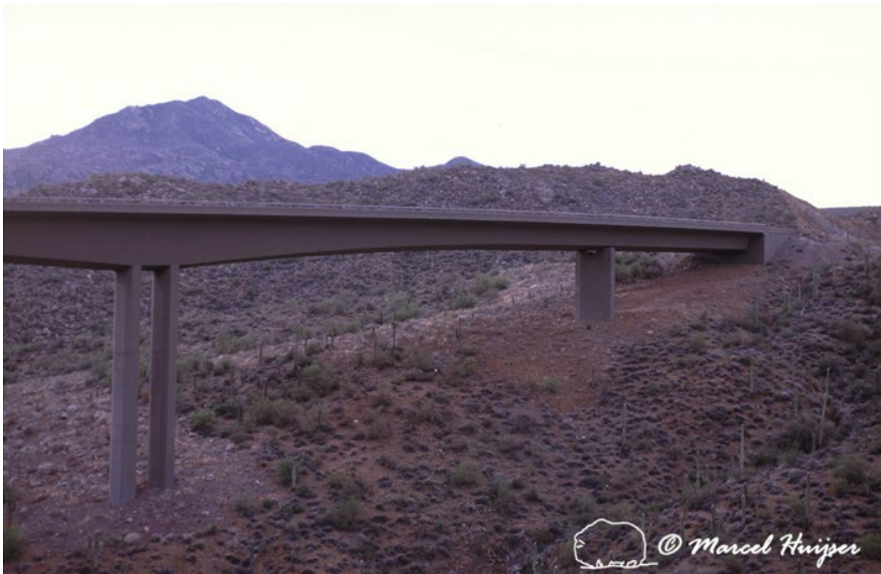
Figure 54. Bridge shortly after construction, Tonto National Forest, Arizona, USA. Note that the impacts of the construction on the vegetation and soil have been minimized.
