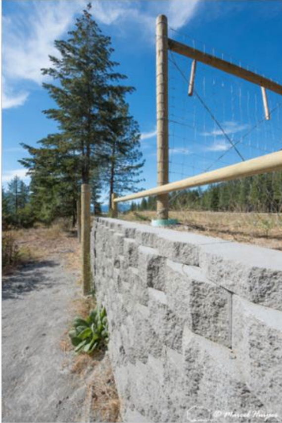
Figure 45. Wildlife jump-out with concrete blocks and a bar for bighorn sheep ( Ovis canadensis ), near Thompson Falls, Montana, USA. Note that it is probably better to not have the concrete blocks protrude as it makes it easier for species to climb the face.
