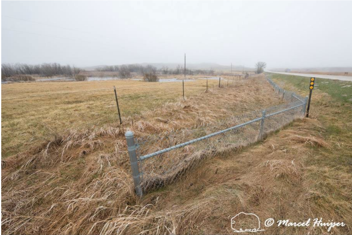
Figure 102. Though not meeting the recommended specifications for a “turn-around fence-end”, this is an attempt at discouraging turtles from crossing the road in high numbers at the fence-end, US Hwy 83, Valentine National Wildlife Refuge, Nebraska, USA.
