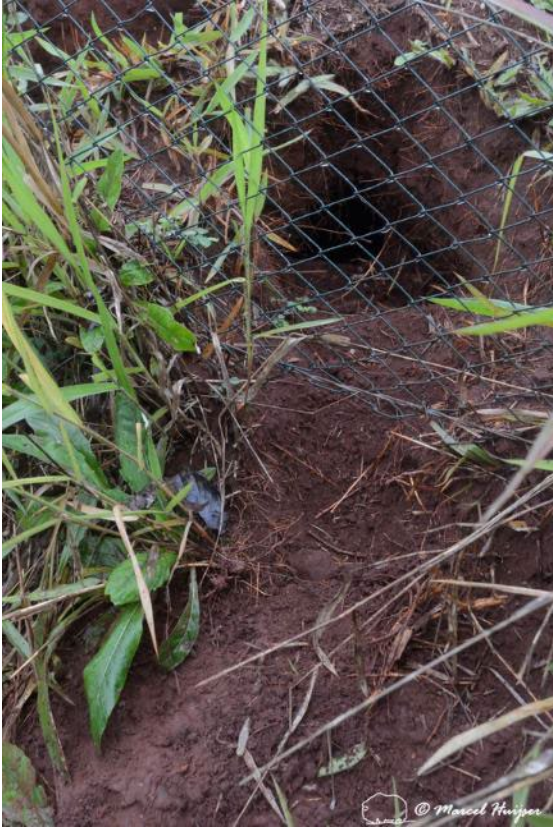
Figure 110. An animal (probably a nine-banded armadillo ( Dasypus novemcinctus )) dug a gap under a wildlife fence. The burrow is visible on roadside of the fence, SP-225 motorway, near Brotas, São Paulo, Brazil.
