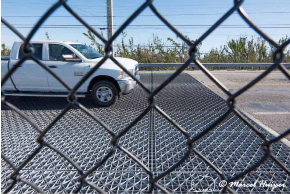
Figure 29. Wildlife guard at a fence-end on US Hwy 1, Big Pine Key, Florida, USA.
