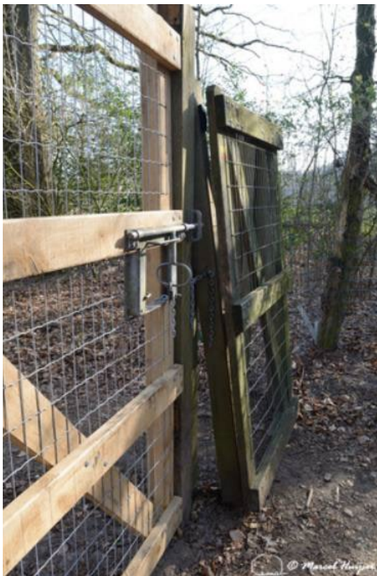
Figure 41. Swing gate at a wildlife fence, set at an angle so it closes through gravity, The Netherlands.
