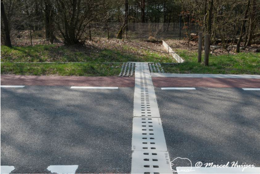
Figure 96. Amphibian tunnel with open slotted roof and barrier or wall for amphibians, integrated into roadbed, Deelenseweg, between Hoenderloo and Arnhem, Gelderland, The Netherlands.
