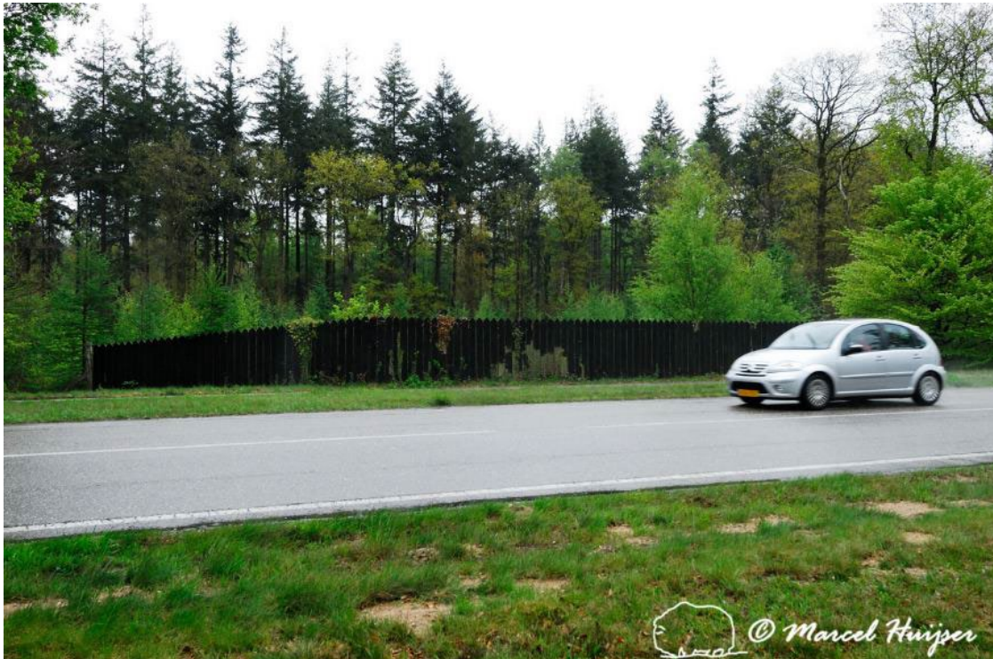
Figure 19. Visual barrier above a wildlife underpass, Amersfoortseweg, Hoog Soeren, The Netherlands. The fence reduces visual and noise disturbance from traffic for the animals that approach the underpass.
