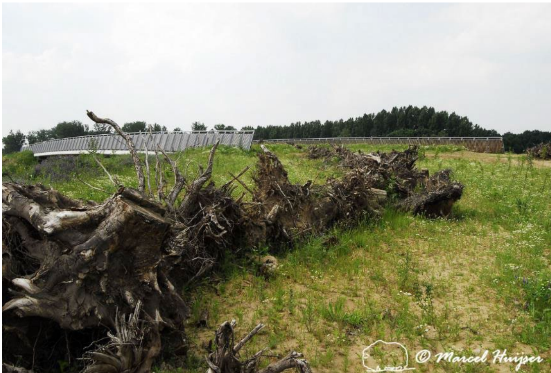
Figure 86. Root wads leading up to and on top of wildlife overpass as cover for small animal species, The Netherlands.
