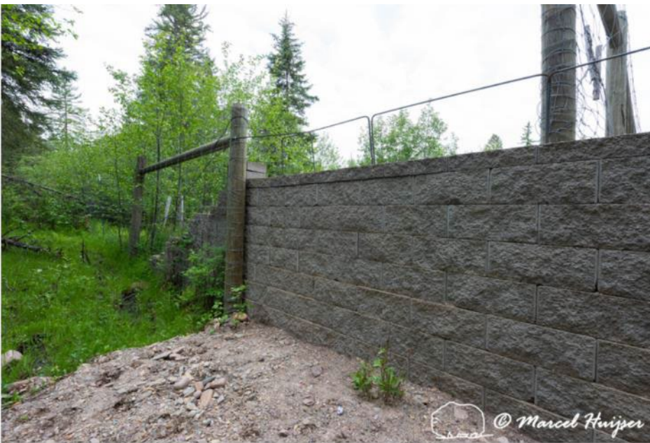
Figure 46. Wildlife jump-out along US Hwy 93, Flathead Indian Reservation, Montana, USA. Jump out is 5 ft tall with rebar on top.
