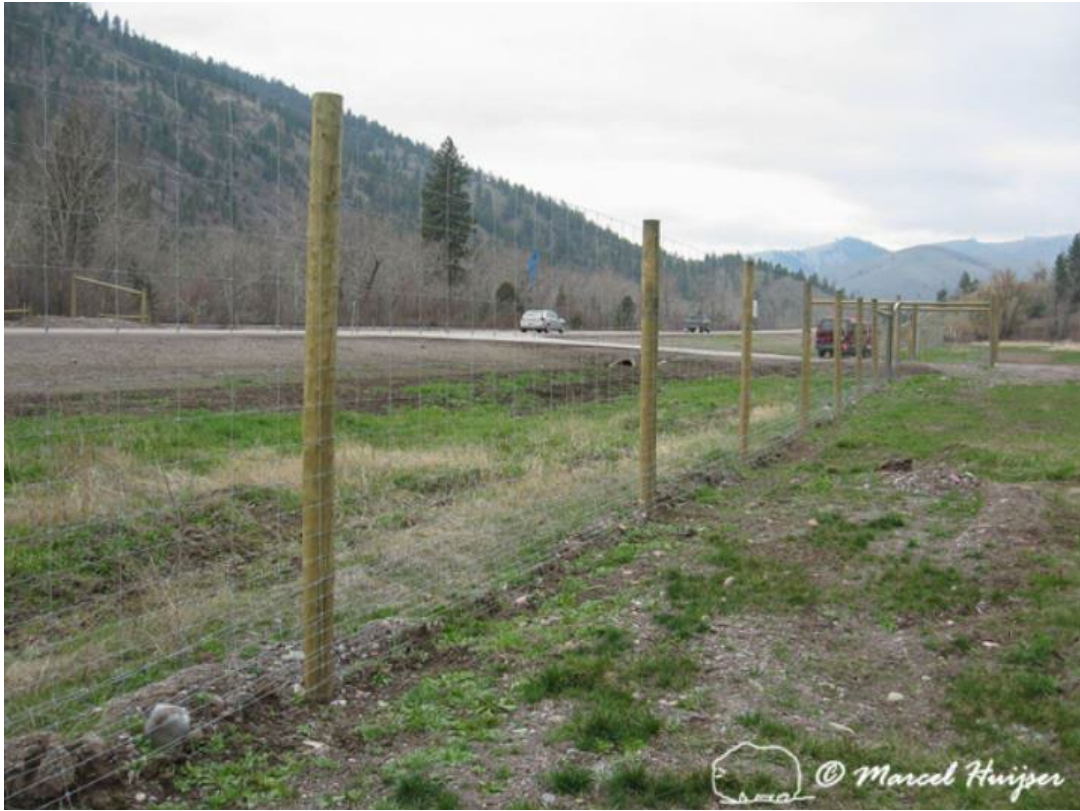
Figure 7. Typical large ungulate fence in North America, 8 ft tall, wooden posts and mesh-wire fence material, US Hwy 93 North, Montana, USA. Note that there is a dig barrier attached to the main fence material (e.g. for canids).
