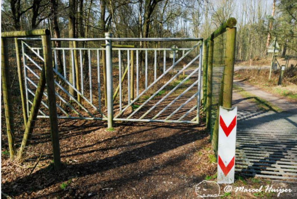
Figure 42. Wildlife guard (right) and horse gate (left), Heugterdijk, Weerterbos, near Maarheze, The Netherlands. The riders do not have to dismount and can push the rotating gate while in the saddle. The gate is set at an angle so that gravity will bring the rotating fence in line with the main fence.
