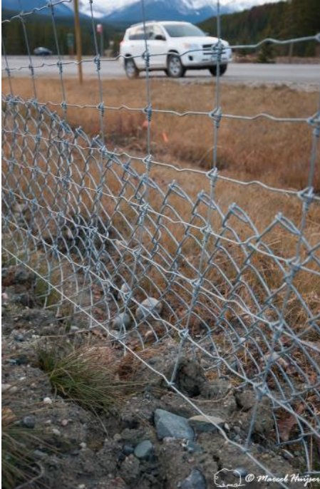
Figure 70. Wildlife fence and dig barrier (or “apron”), mostly for canids and bears ( Ursus sp.), Trans-Canada Highway, Banff National Park, Alberta, Canada. The dig barrier angles away from the road and keeps the animals from digging under the fence.
