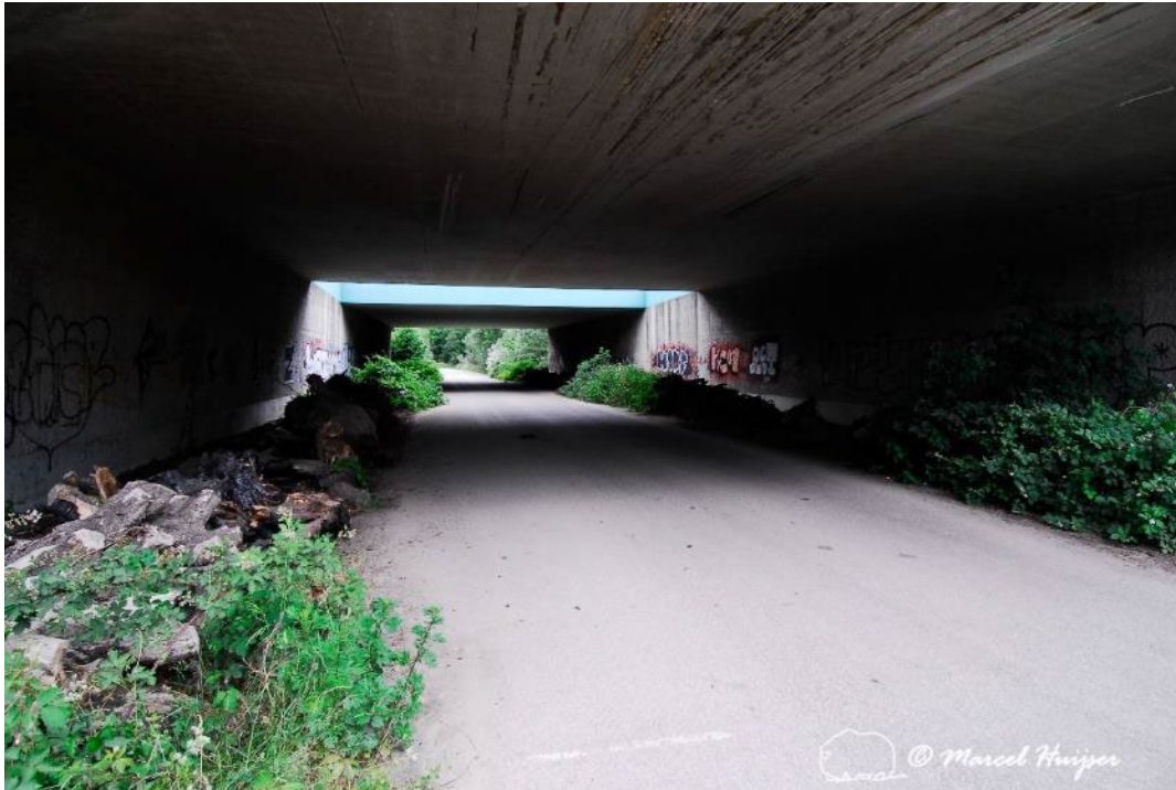
Figure 99. An existing underpass for a low volume road under a 4-lane A27 motorway, near Hilversum, The Netherlands. The structure was made more suitable for small animal species by placing rows of root wads along the sides.
