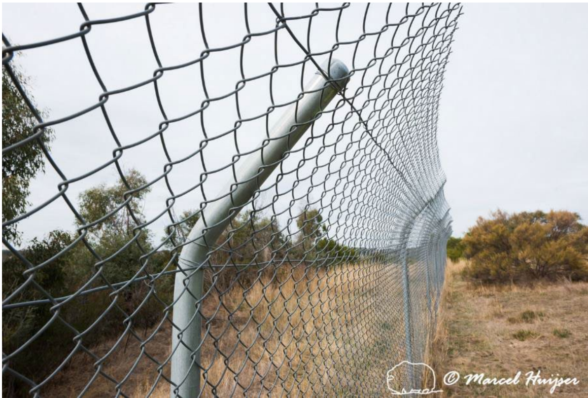
Figure 74. Fence designed to keep koala ( Phascolarctos cinereus ) off the highway, M79, between Harcourt and Faraday, Victoria, Australia. This fence is about 2.1 m high, and the top 50 cm or so angles away from the road. The last 30 cm or so is not supported by the post and forms a ‘floppy top’ making it difficult to cross by species that climb well.
