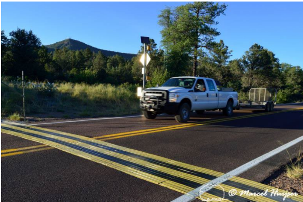
Figure 30. Electrified mat associated with an animal detection and driver warning system at a fence-end, S.R. 260 east of Payson, Arizona, USA.
