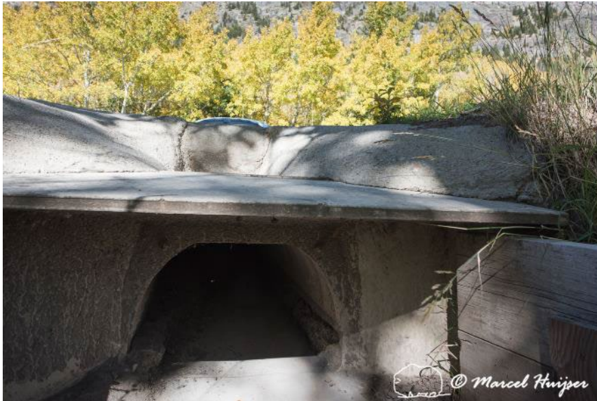
Figure 83. Culvert for long-toed salamander ( Ambystoma macrodactylum ), Waterton Lakes National Park, Alberta, Canada.
