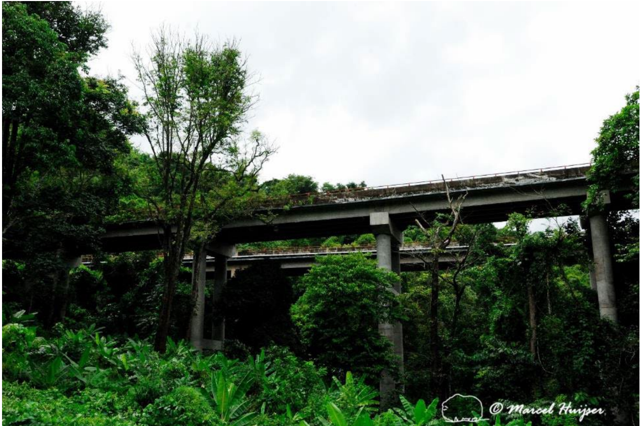
Figure 87. Tall bridges allow for light and moisture under the structure, and for continuous habitat for nearly all species, including small animal species, China.
