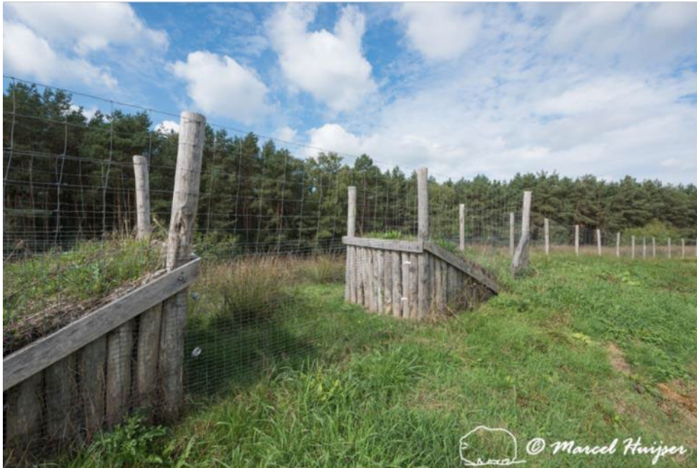
Figure 49. Wildlife fence and jump-out along A28 motorway, near Spier, Drenthe, The Netherlands. The fence is a barrier for medium and large mammal species. The electric fence is an additional barrier for livestock (sheep, cattle) that are used as a tool for nature management in the area.
