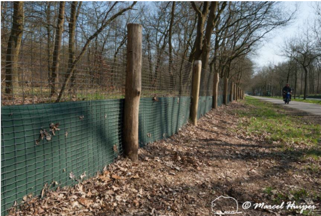
Figure 61. A “fence” designed for Eurasian badger ( Meles meles ) (the taller metal fence material with small mesh size) and for common toad ( Bufo bufo ) (the plastic sheets at the bottom of the fence), Rijksstraatweg Elsterstraatweg N225 just west of Elst, Utrecht, The Netherlands.
