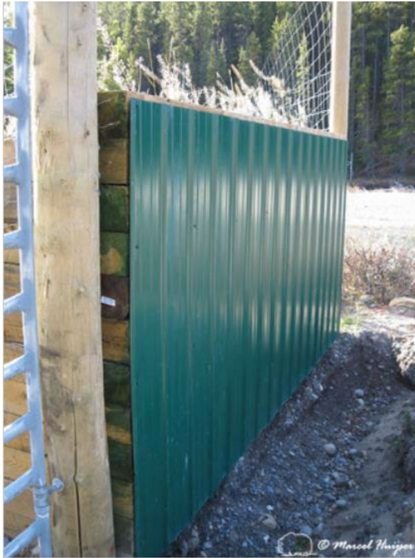
Figure 47. Wildlife jump-out with a smooth metal face to reduce the likelihood that bear will climb the jump-out and end up in fenced right-of-way, Banff National Park, Alberta, Canada.
