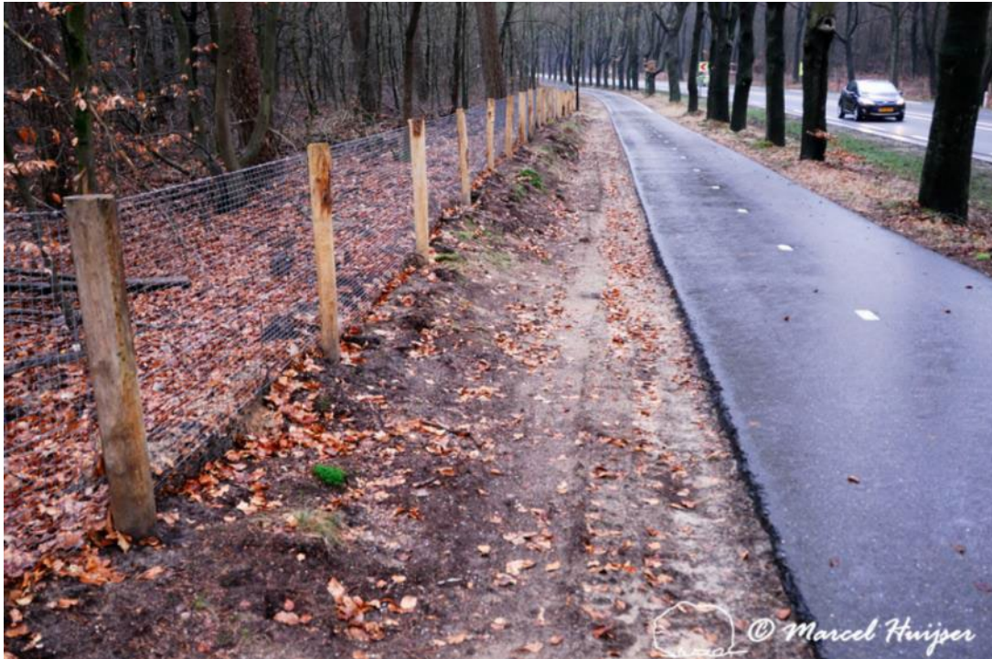
Figure 63. Wildlife fence for Eurasian badger ( Meles meles ) and wild boar ( Sus scrofa ), N302, Leuvenumseweg, Sonnevank, east of Harderwijk, The Netherlands.
