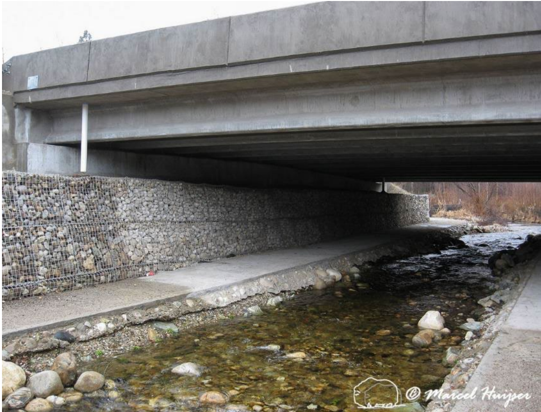
Figure 92. Pathway for large mammals in an underpass (bridge) primarily designed for water (stream), US Hwy 93 S, Bitterroot Valley, Montana, USA.
