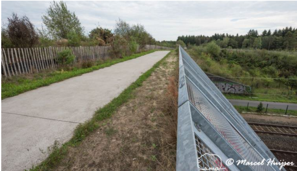
Figure 22. Hiking and biking trail combined with wildlife overpass across railroad tracks, Soest, The Netherlands. The “wildlife area” on the overpass is further to the left, separated from the trail by a berm and shrubs and trees.
