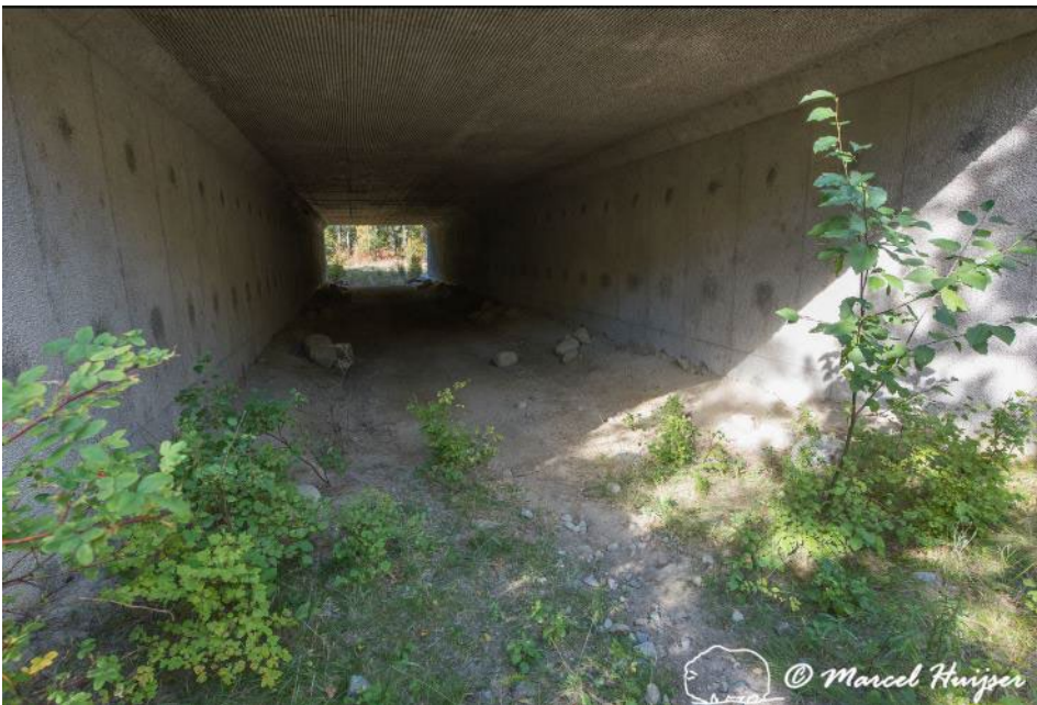
Figure 89. Vegetation providing cover at the approach of a wildlife underpass, US Hwy 95, Bonners Ferry, Idaho, USA.
