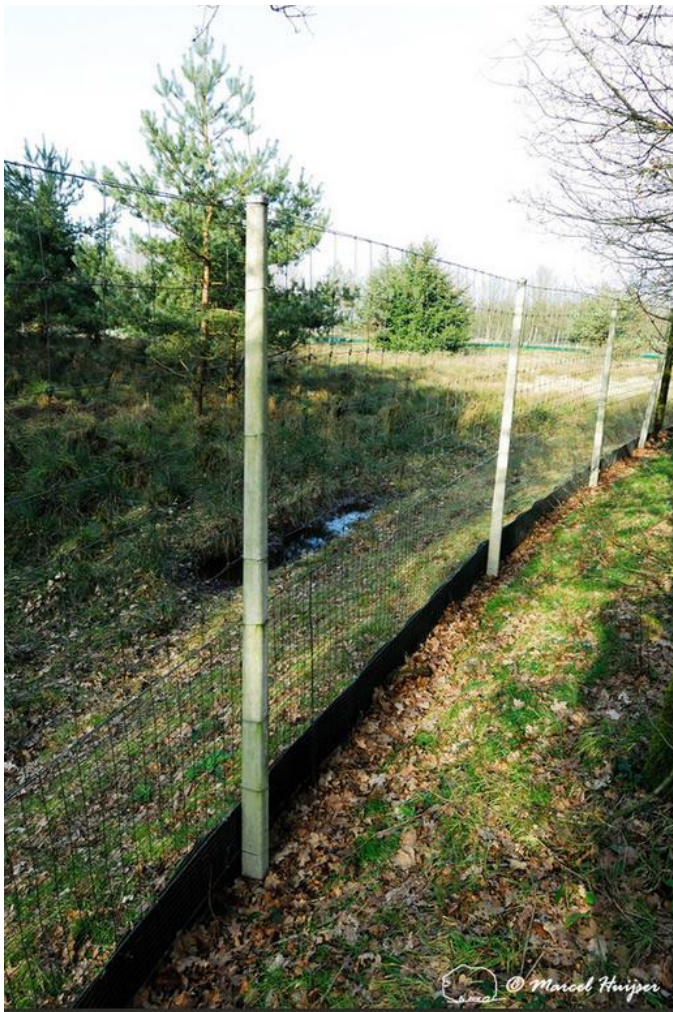
Figure 12. Wildlife fence for amphibians (e.g. common toad ( Bufo bufo )), medium sized mammals (e.g. Eurasian badger ( meles meles )) and large ungulates (e.g. roe deer ( Capreolus capreolus ), red deer ( Cervus elaphus )) at ecoduct Woeste Hoeve A50 near Apeldoorn, The Netherlands.
