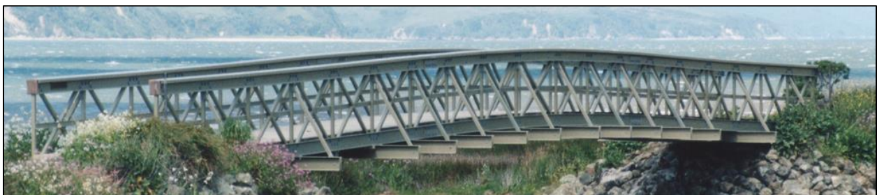
Figure 3: Example of pultrusion-style pedestrian bridge in Marshall, CA. Bridge spans 29 m and is 1.8 m wide. With a live-load design of 2.83 kilopascals (kPa), or 60 pounds per square foot (psf), the FRP members are connected with galvanized steel bolts [18].
