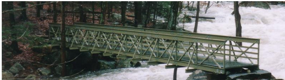
Figure 11: Example of a pedestrian bridge built by Creative Pultrusions. This bridge is in Bear Mountain, New York, and is 62ft x 6ft with a straight design using FRP railings for trusses and FRP decking for the walkway.
