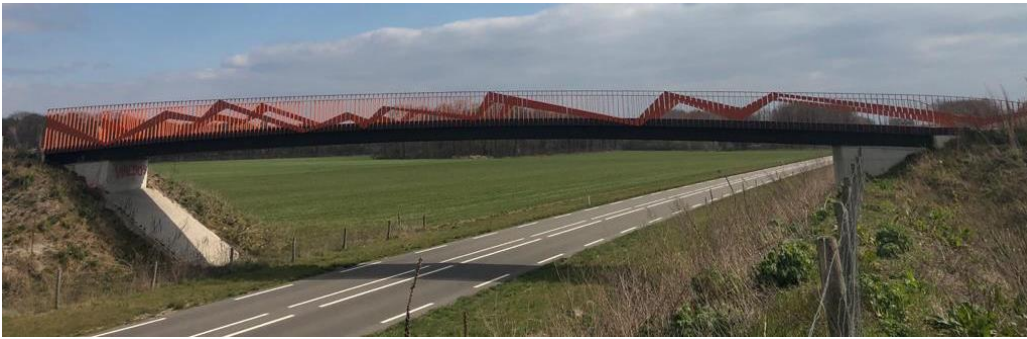
Figure 19: The longest, unsupported, uni-mold bridge built by FiberCore Europe using InfraCore® technology. The bridge is 37m x 3.5m and has a design-load of 5kN/m 2 (~104psf).
