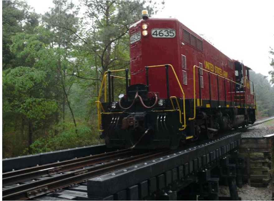
Figure 20: Pultrusion-style train bridge built from recycled plastic. Axion Structural Innovations created two spans of 40ft and 80ft that can support 130-ton locomotives.
