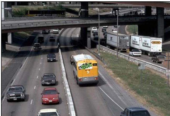
Figure 1-3: A Contraflow Lane Using a Moveable Barrier
