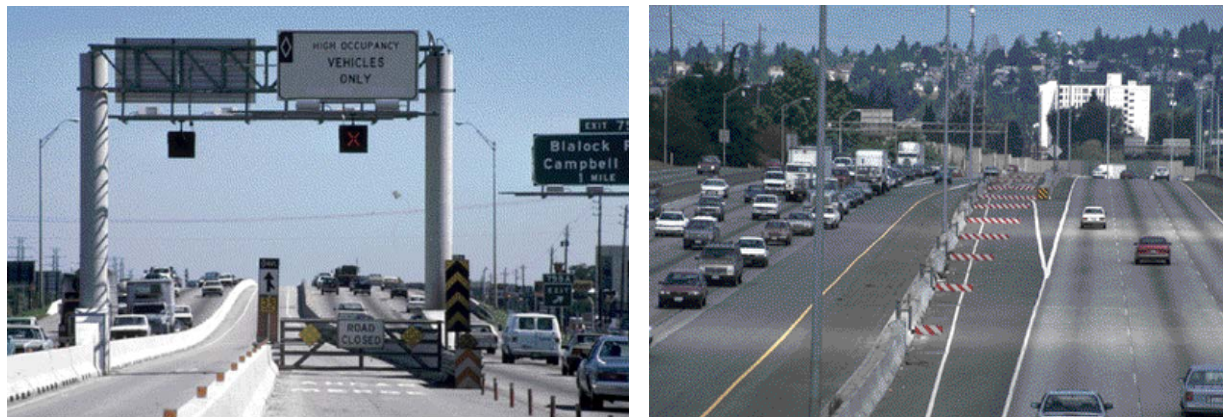
Figure 1-4: Channelized Access for Reversible-Flow Lanes
