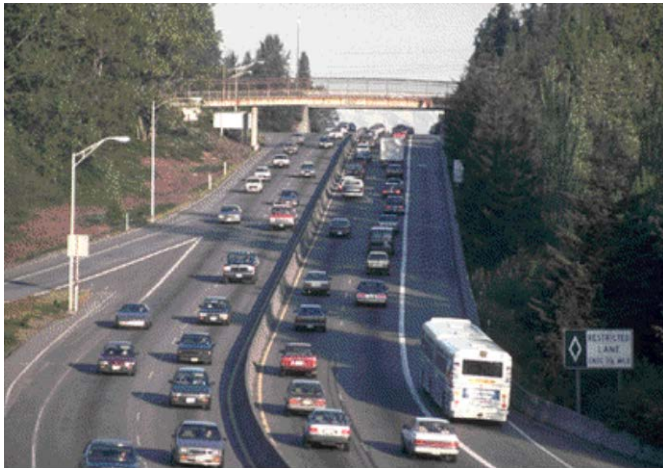
Figure 1-16: Right-Side HOV Lanes Operated on Shoulder
