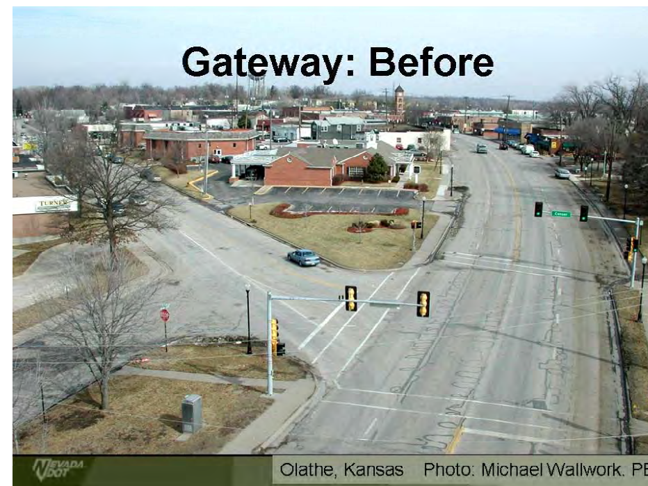
Figure 4-6 Signalized Intersection in Olathe, Kansas before Roundabout is Installed
