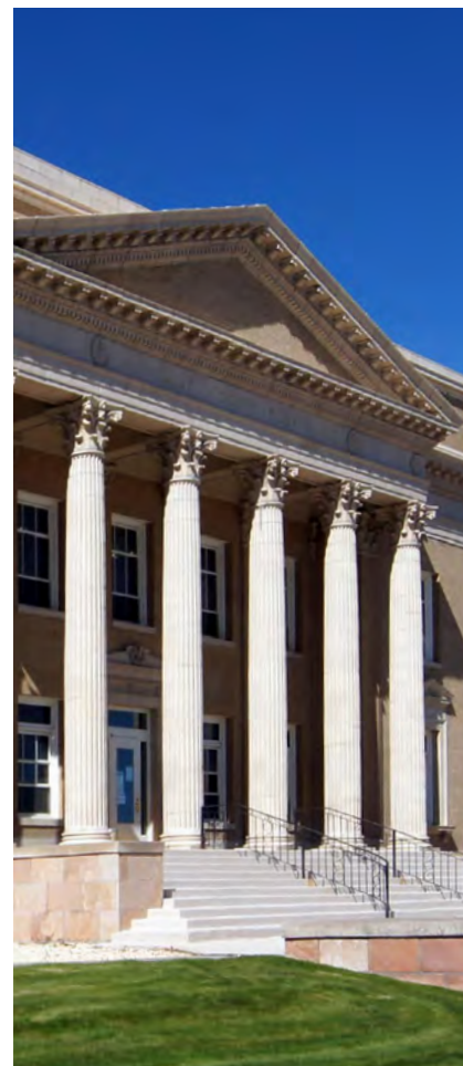
▲ The Sixth Judicial District Court is located in the Humboldt County Courthouse in Winnemucca.
