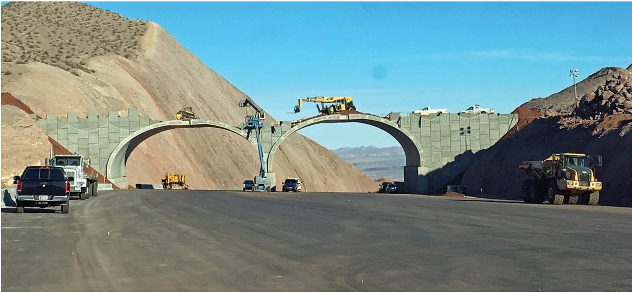
*Installation of BEBO arches during construction of I-11 crossing*
