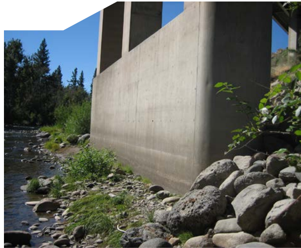
Existing piers located within 100-year floodplain.
