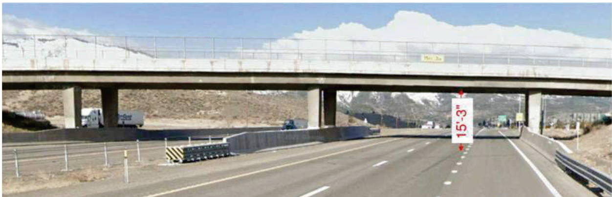
View of I-770 existing vertical clearance at 15'-3". The minimum required clearance by today's standards is 16'-6".
