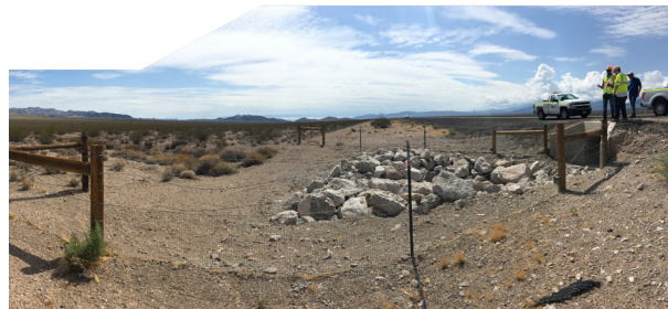
Drainage Structure/Crossing and Fencing.
