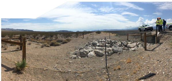
Drainage Structure/Crossing and Fencing.
