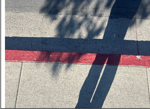
Red Paint on Concrete Curb
