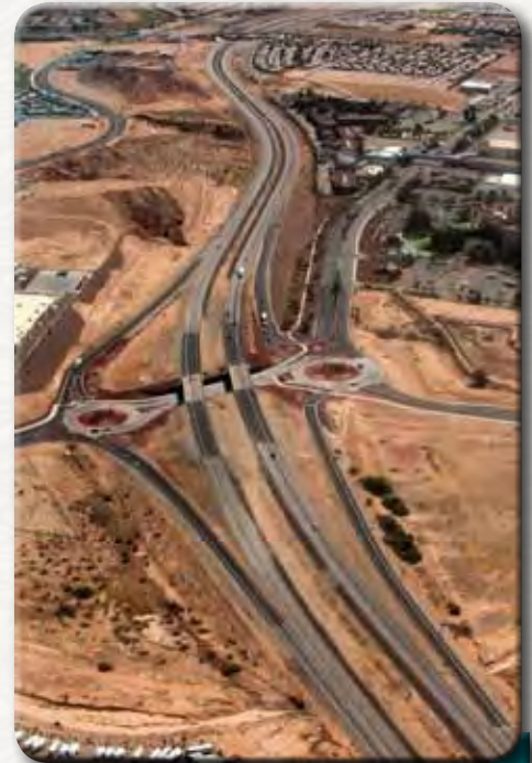
Work completed on the new bridges at the West Mesquite Interchange.
