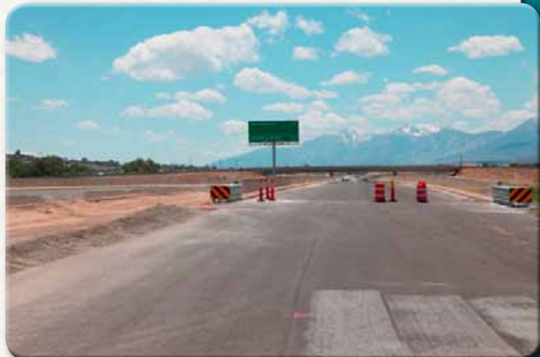
US 395 fm South Carson St to Fairview Dr. Carson City
