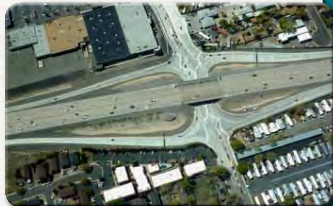
Aerial view of the completed Moana Lane Diverging Diamond Interchange.
