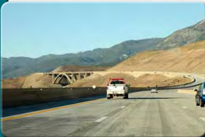
The Galena Creek Bridge as seen heading south on the I-580 freeway extension.
