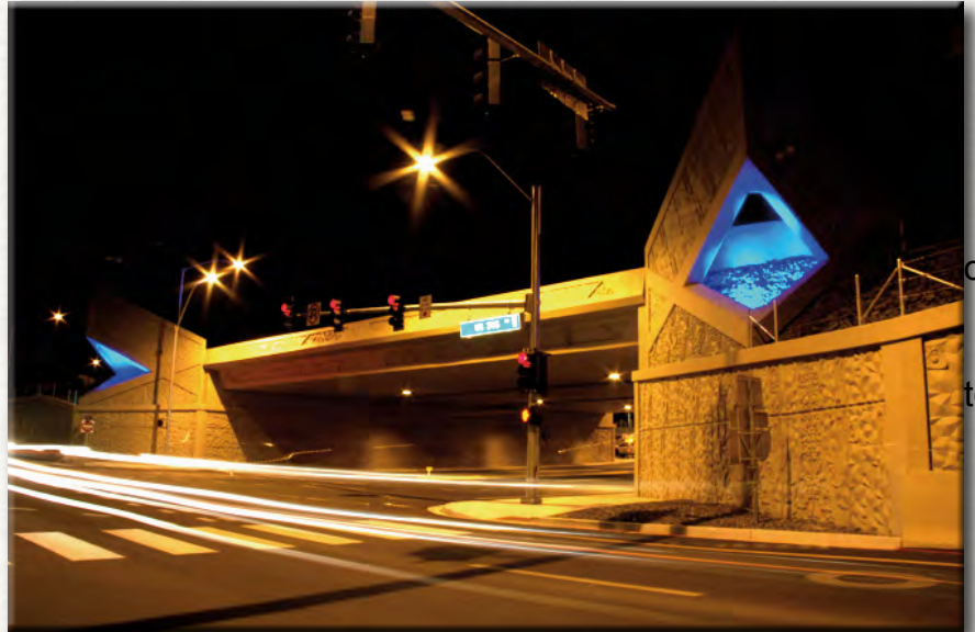
Aesthetic additions to a bridge structure lit with color changing LED lights for the I-580/ Meadowood project. @Vicki Scuri 2013, Courtesy of Vicki Scuri Siteworks
