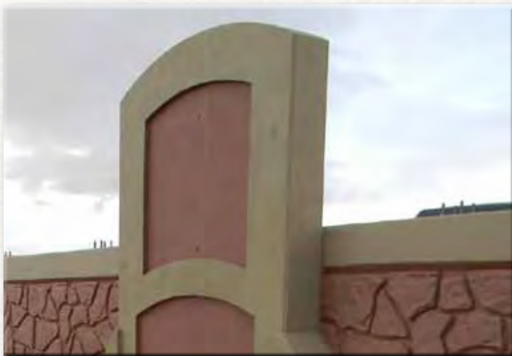
Integrating aesthetics with the Route 766 bridge on I-80 in Carlin.
