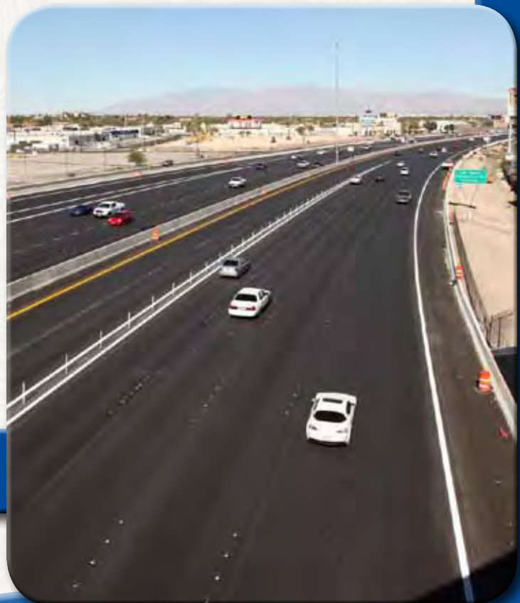
Asphalt rubber improves Interstate 15 through the heart of Las Vegas.
