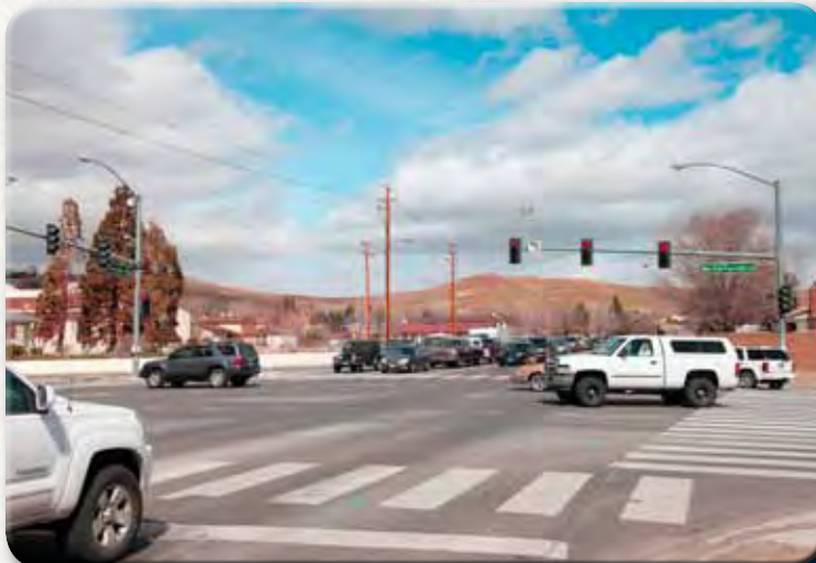
SR 445 Pyramid Highway at North McCarran Blvd Reno
