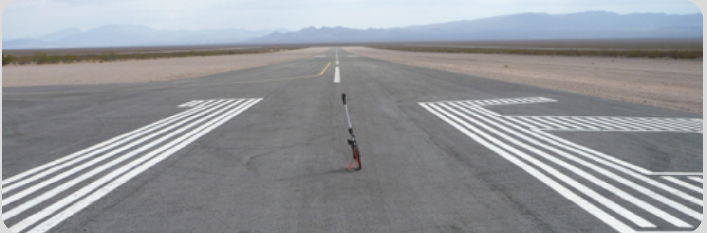
Nevada Statewide Airport Pavement Summary.
