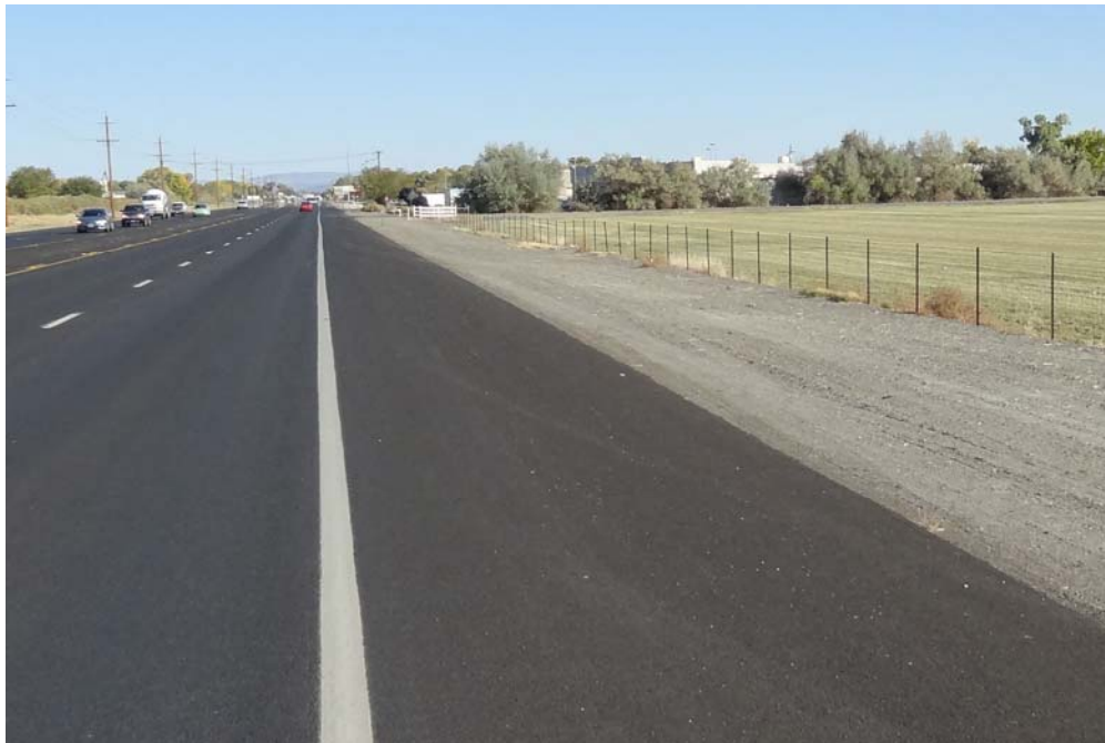
Figure 7 – Paved Shoulder Facility
