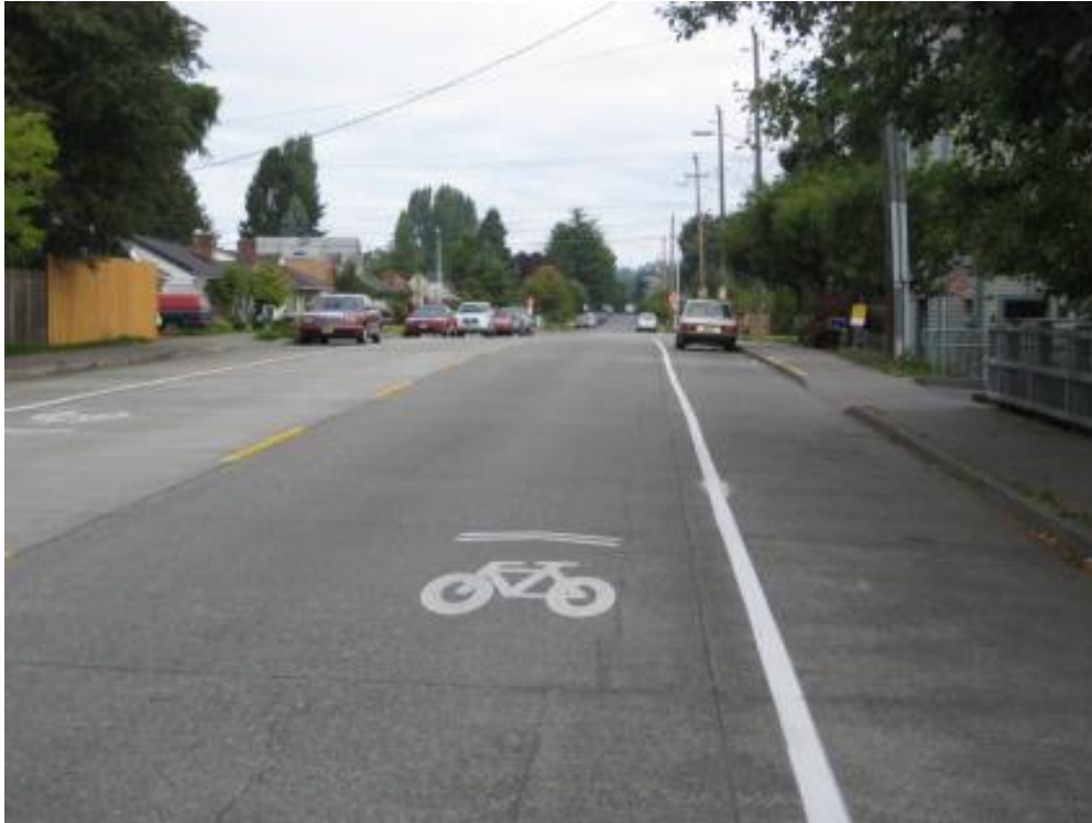
Figure 5 – Marked Shared Lane Facility
