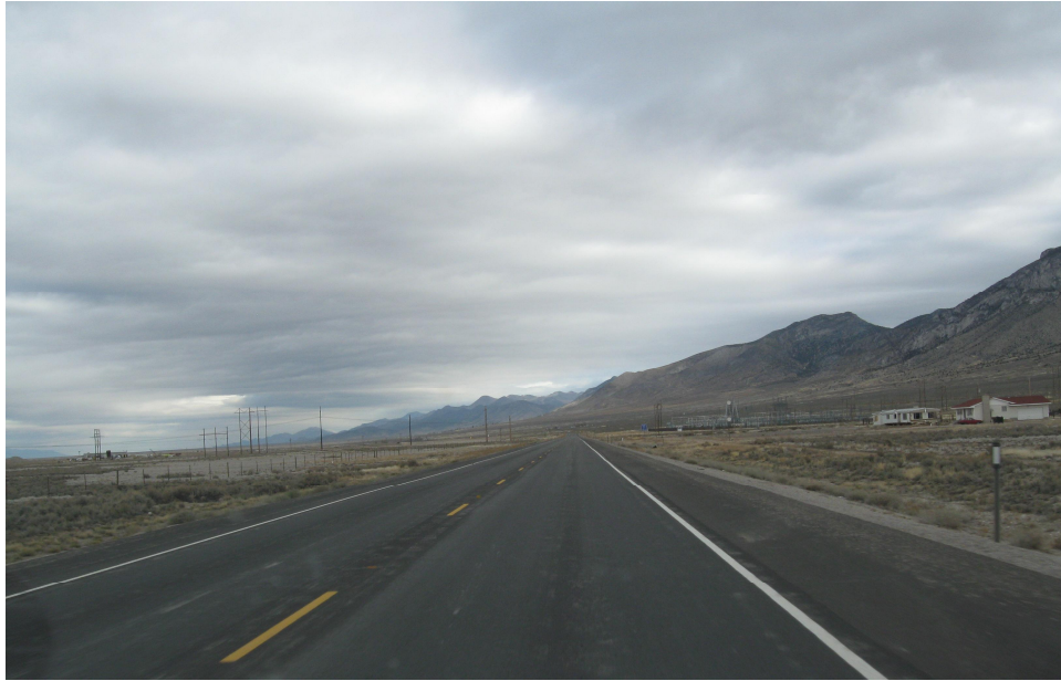
Figure 6 – Paved Shoulder Facility
