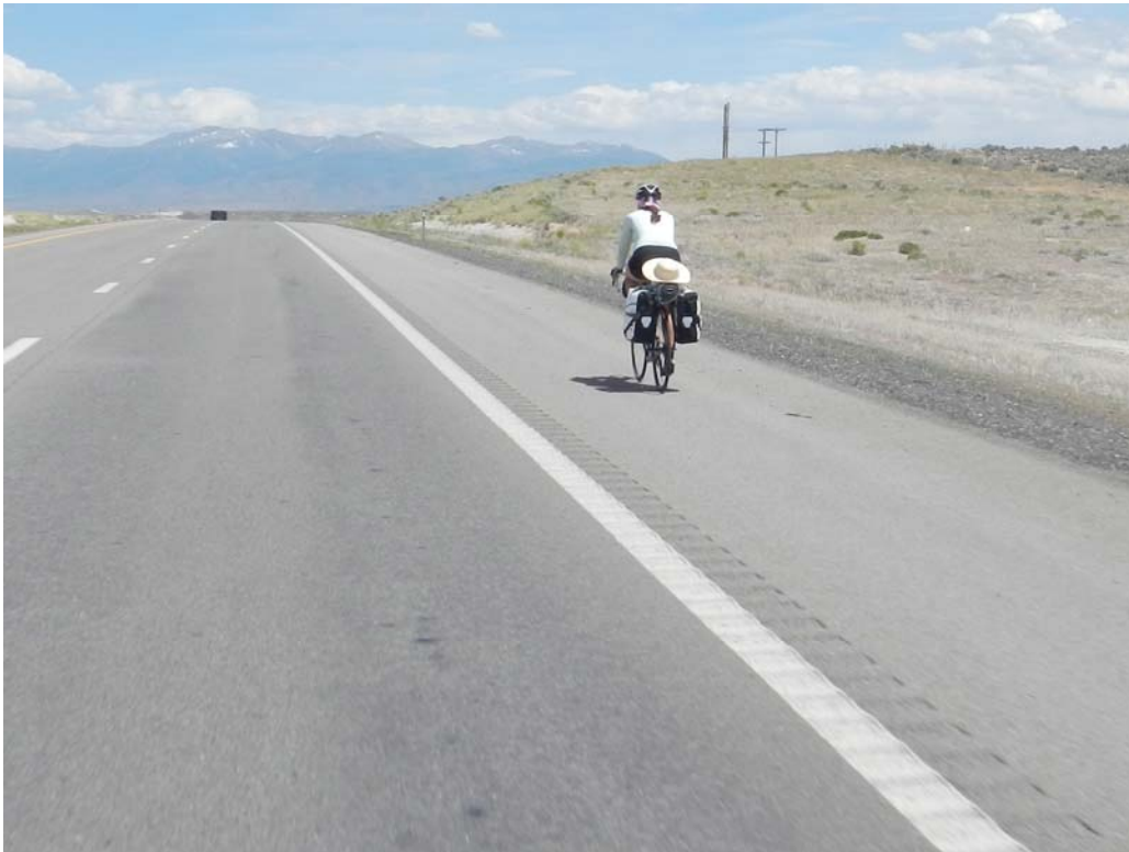
Figure 4 – Paved Shoulder Facility
