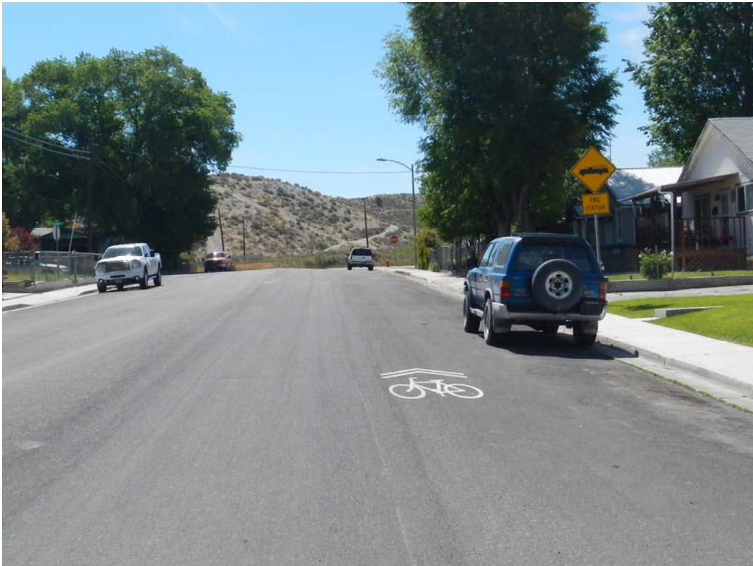
Figure 3 – Marked Shared Lane Facility
