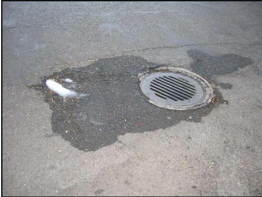
Figure 1-34. Residual foam and dampness around an inlet suggests potential illicit dumping. (Photo by T. Svetich)
