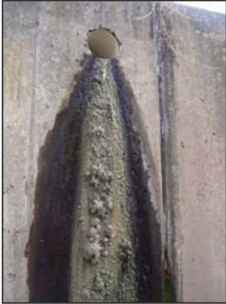
Figure 1-29. This excessive algae growth suggests a discharge high in nutrients that may or may not be illicit. (Photo from the Chesapeake Stormwater Network)
