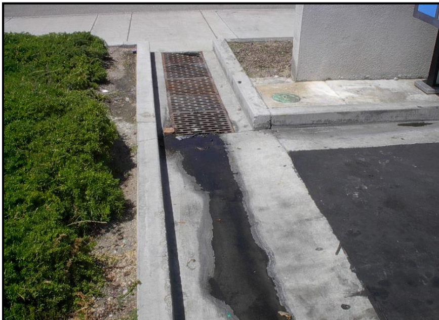
Figure 1-15. An unusual, black discharge flows to the storm drain. (Photo from the USEPA)
