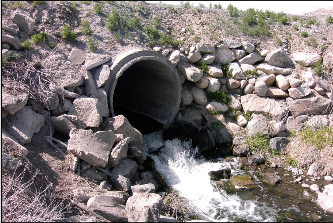
Figure 1-10. This photo shows a flowing outfall, but there was no recent rain fall (notice the ground is dry). (Photo from the City of Reno)
