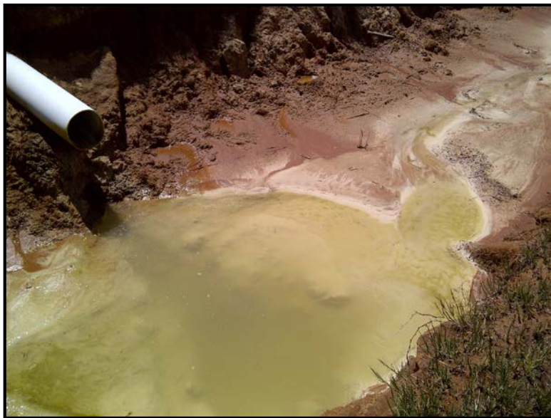
Figure 1-30. This photo shows a “dead zone” at the outfall due to the possible discharge of a toxic chemical. (Photo from GUBICO)
