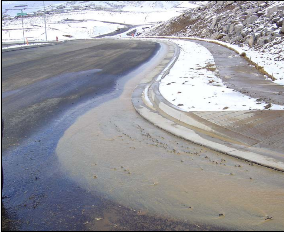
Figure 1-9. Sediment discharge into the MS4 from an unstabilized cut slope with no BMPs would be considered “indirect” and “transient”. (Photo from the City of Reno)
