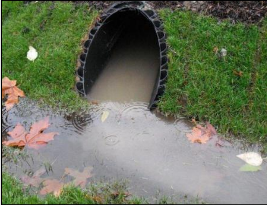
Figure 1-16. This photo shows a brown discharge at an outfall that is likely the result of sediments. (Photo from the Washington State Department of Transportation)
