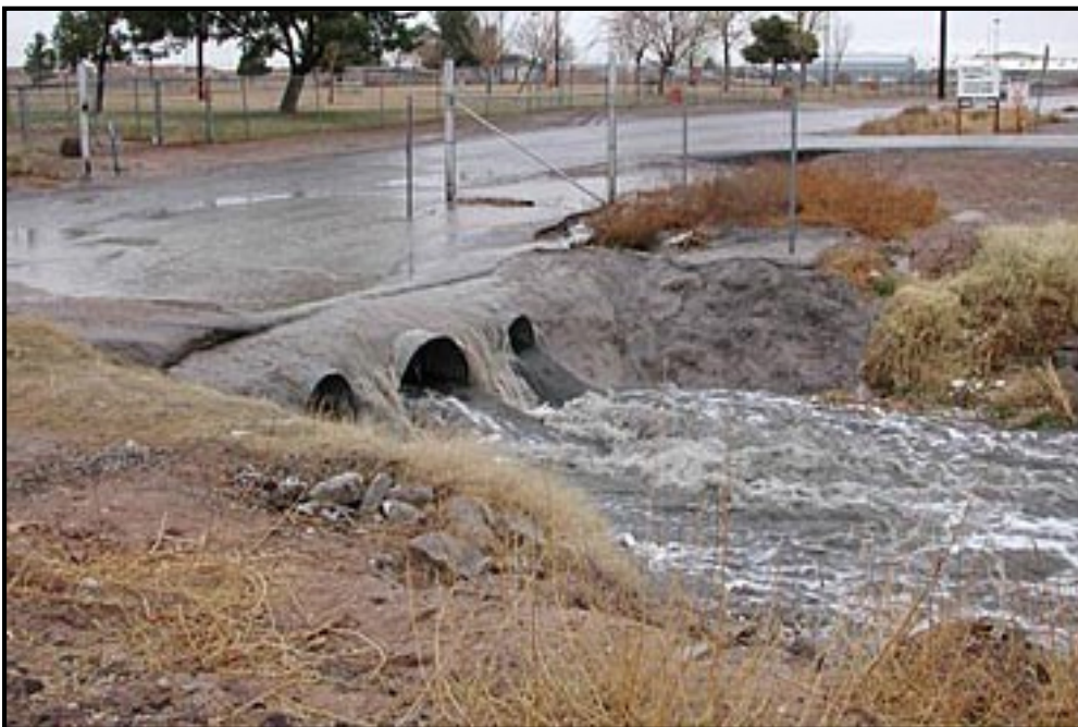
Figure 1-11. The outfalls shown in this photo are flowing strongly after a rain event. (Photo from the Tahoe Environmental Research Center)
