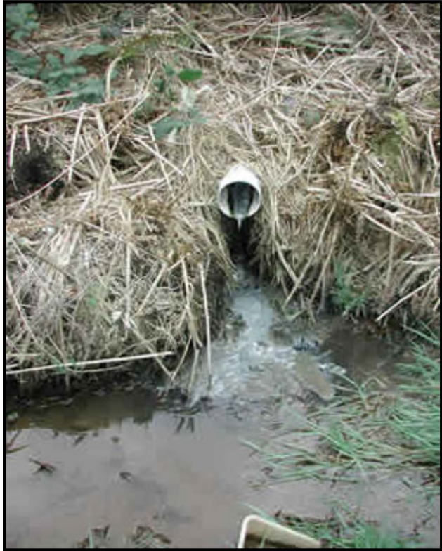
Figure 1-14. This photo shows a gray discharge at an outfall that has the appearance of sewage. (Photo from the Center for Watershed Protection)
